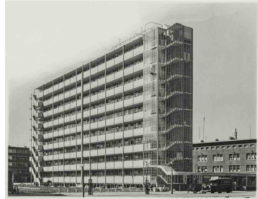
Figure 1: Bergpolderflat in Rotterdam by Van Tijen and Van der Vlugt in 1932
