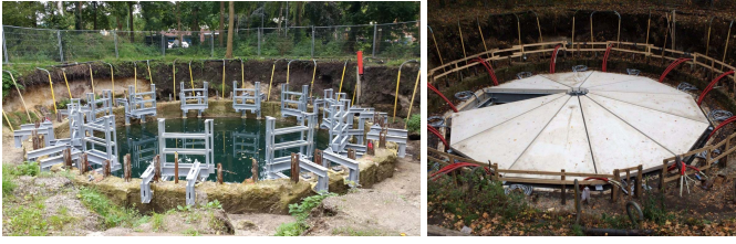
Fig. 2. Construction of the STESS. Left: installation of the last heat buffer. Right: STESS almost completely sealed.
