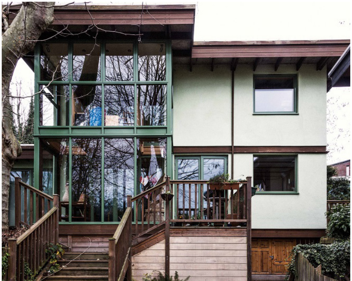
FIG 42. Walter's Way self-build timber housing
