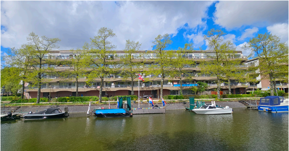
FIG 54. Existing building chosen for intervention
