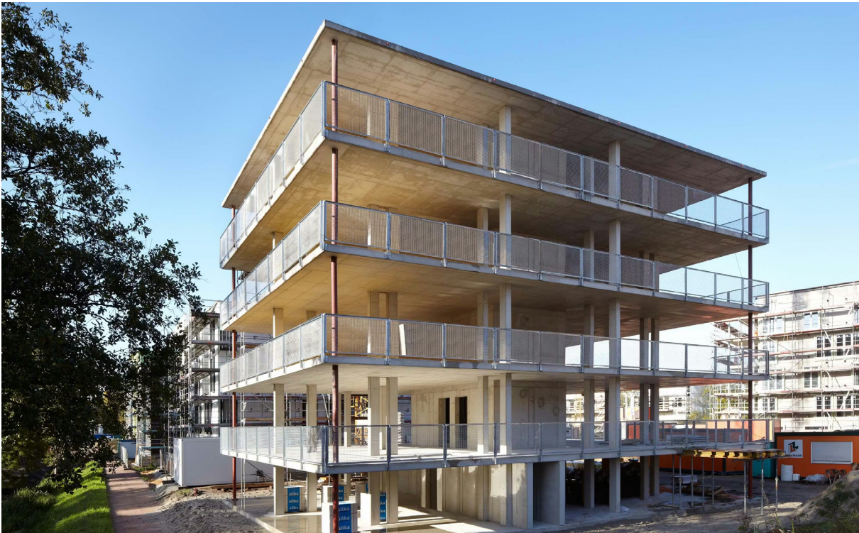
FIG 20. Mach's doch selbst during initial construction phase
