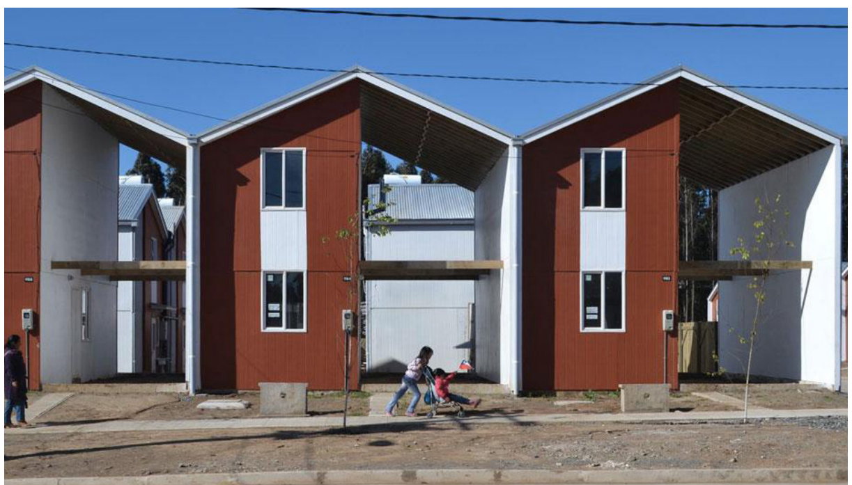
FIG 11. Completed Villa Verde housing units
