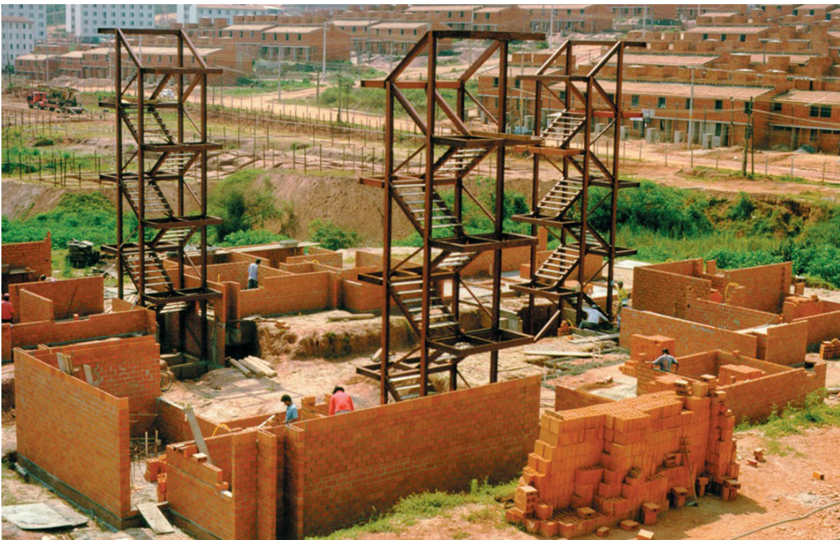
FIG 32. Mutirão construction process
