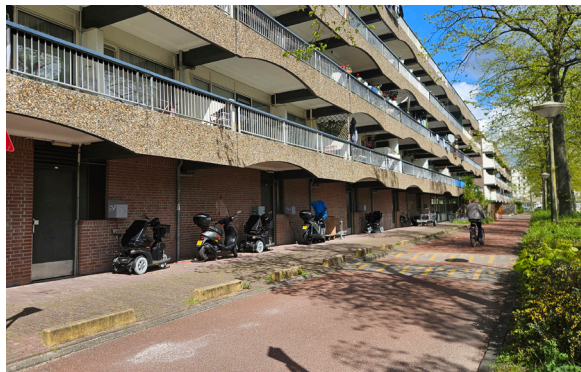
FIG 51. Inactive ground-floor frontage
