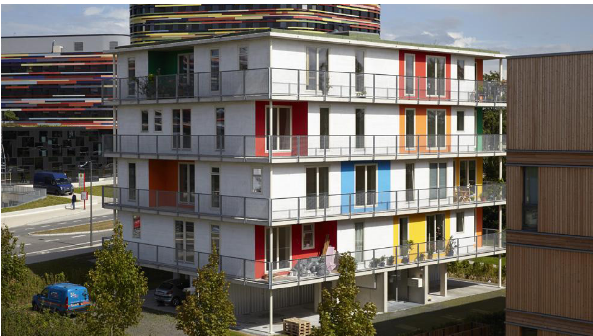
FIG 21. Completed housing block
