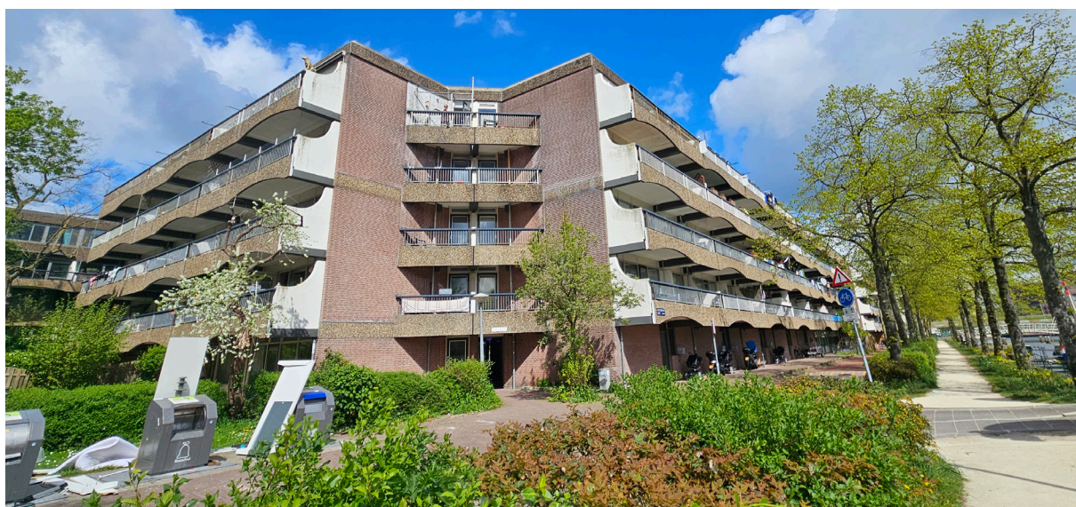
FIG 59. View of building's corner
