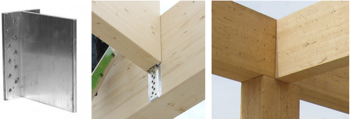
FIG 108. Photos of steel plates connections
