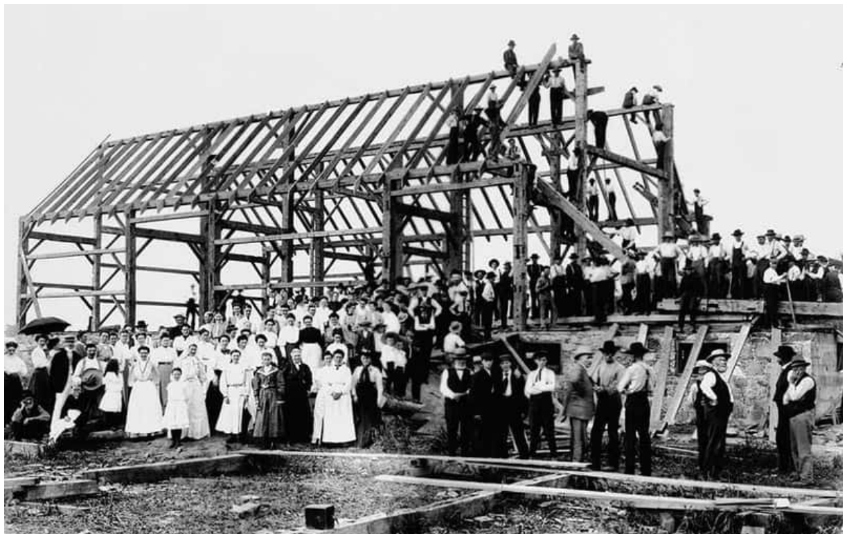
FIG 06. Collective timber construction of a barn in Ontario, Canada, during the 20th century
