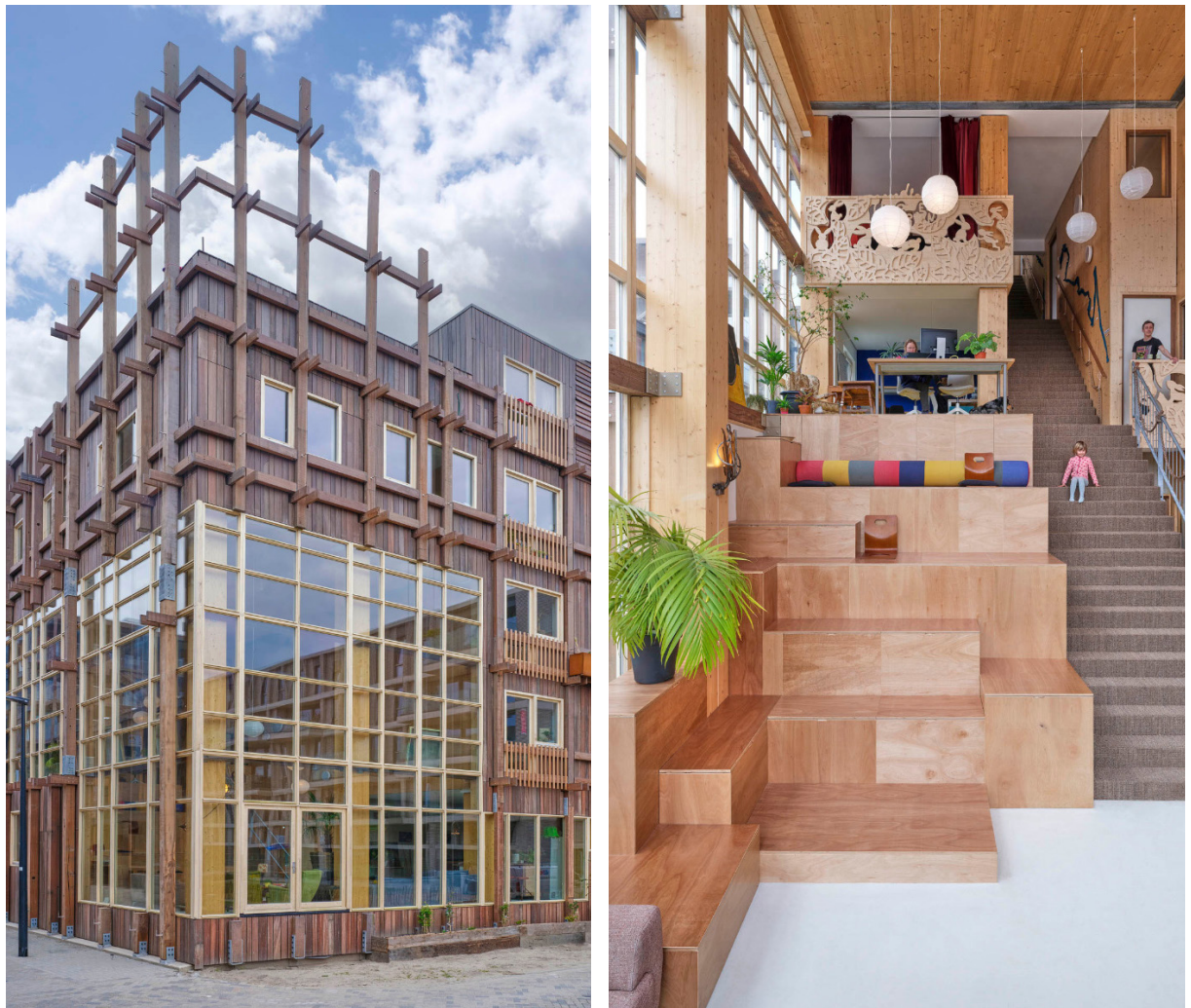
FIG 26. Exterior and communal interior spaces of De Warren
