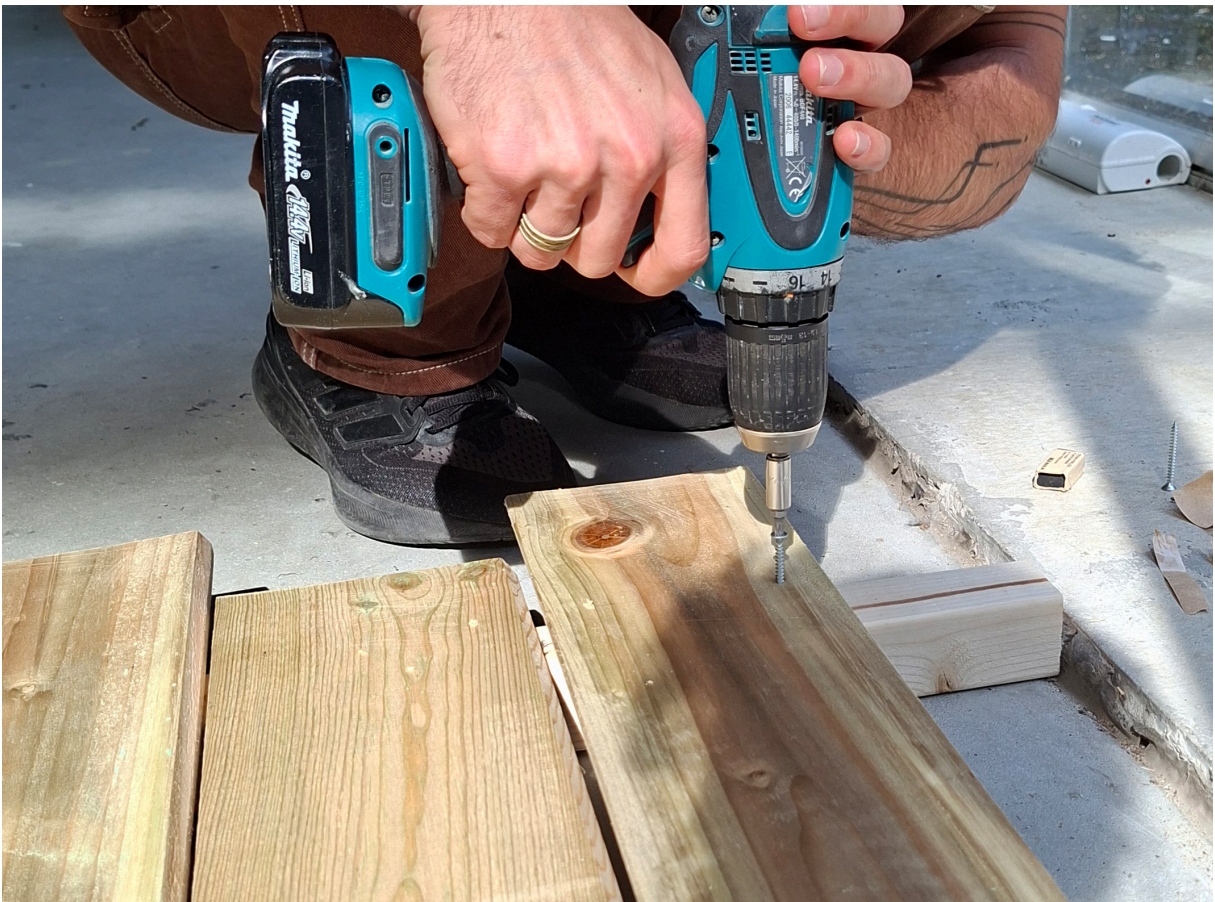
FIG 76. Construction process: physical model open joint horizontal cladding (1:1 scale)
