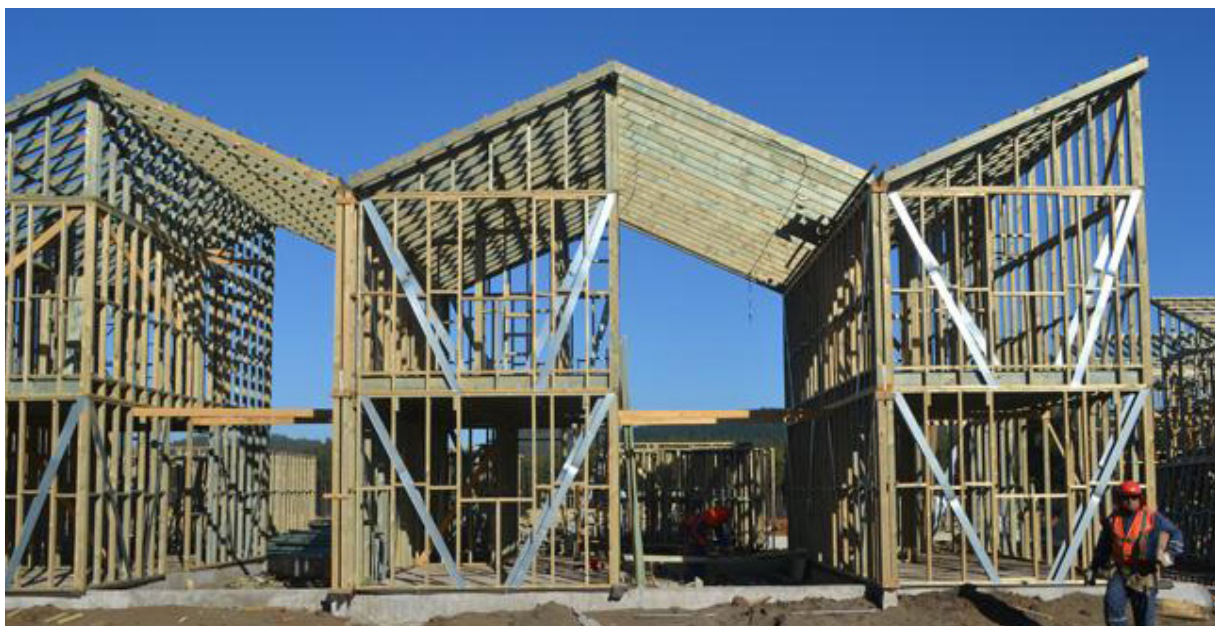
FIG 10. Villa Verde structural timber framework during construction
