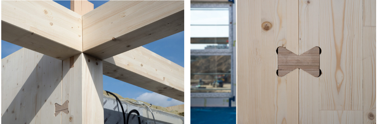
FIG 18. Traditional timber joinery detail
