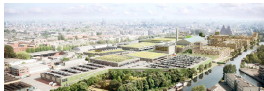
Northern, industrial part of the food centre (VolkerWessels Vastgoed/Ballast Nedam)
