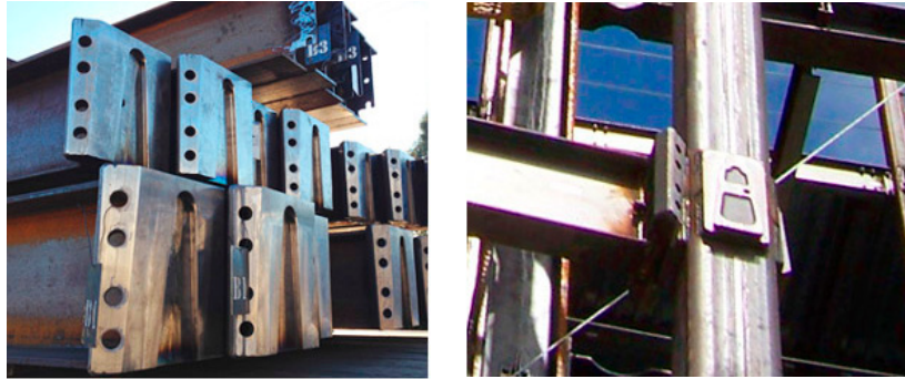
Figure 3.19. Left: ConX beam with shop-welded collar plates Right: Column with shop-welded collar plate (source: http://www.conxtech.com/ , last visited: January 2014)
