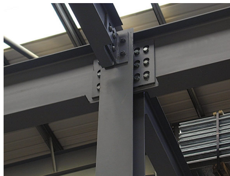
Figure 3.18. Quicon connection applied on an IKEA building (source: http://www.newsteelconstruction.com/wp/quicon-wins-contract-at-ikea/ , last visited January 2014)
