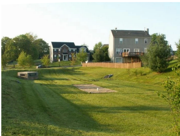
Figure 27. Dry Pond with Sand Filter ( www.ecodesigns.com )
