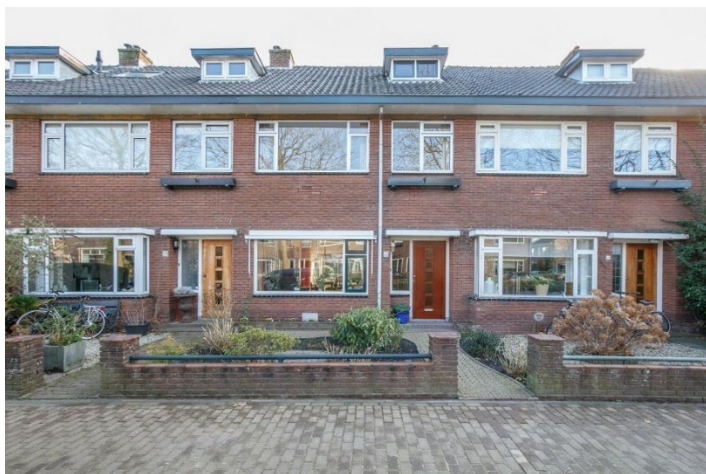
Figure 9 - Terraced house front facade. (funda)
