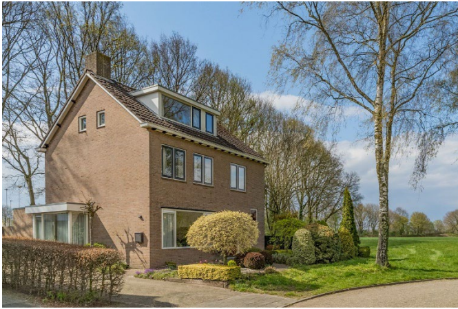
Figure 14- Detached dwelling front façade (funda)
