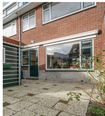
Figure 10 - Terraced house back façade (funda)
