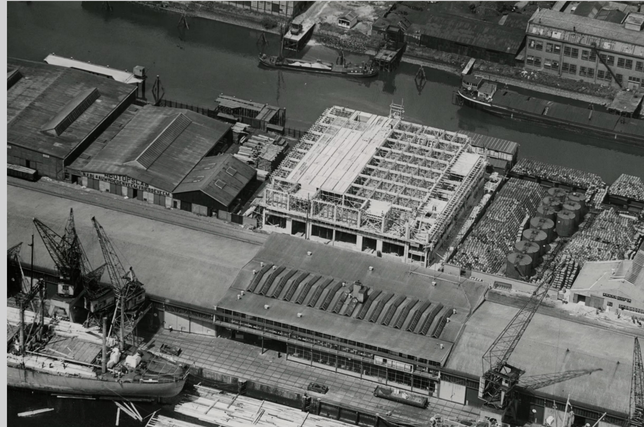
Katoenhuis under construction (1950)
