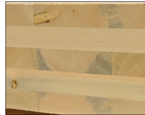
Structural slabs - Cross-lam panels
