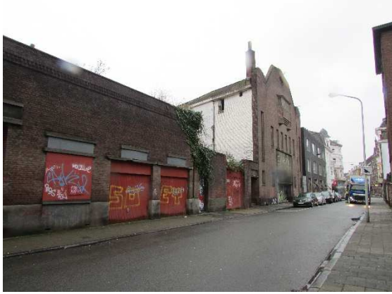
Fig 7 Lage Barakken, buildings to be demolished (own photograph)
