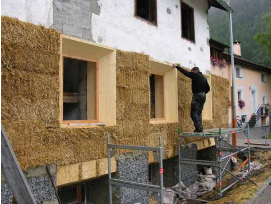
Fig. 8 Insulating with straw - bio-based alternatives for futureproofing buildings. 30
