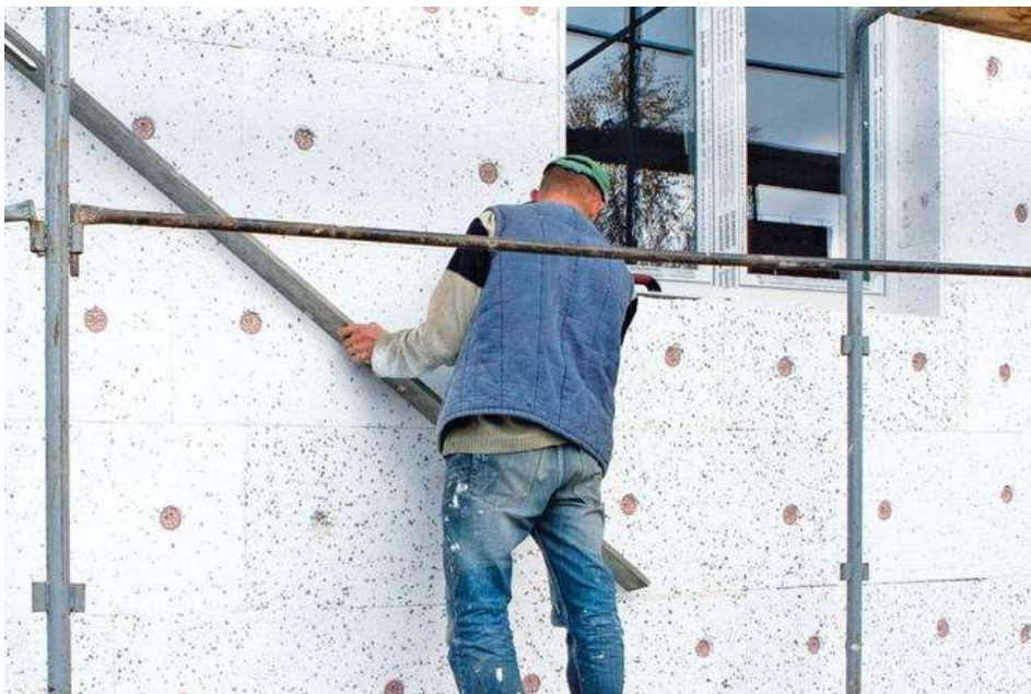
Fig. 7 Adding Styrofoam insulation - Standard practice in Poland. Murator.pl 29
