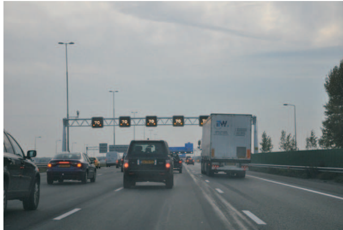
Figure 3.3: Variable Speed Limit Signs
