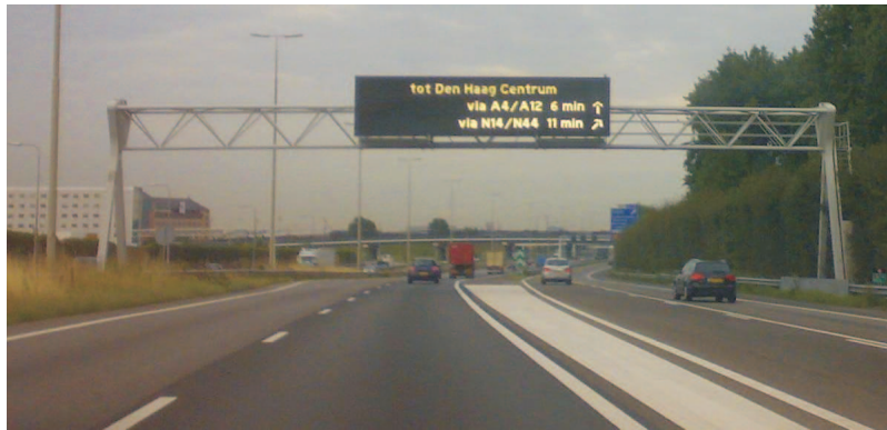
Figure 3.2: Variable Message Sign
