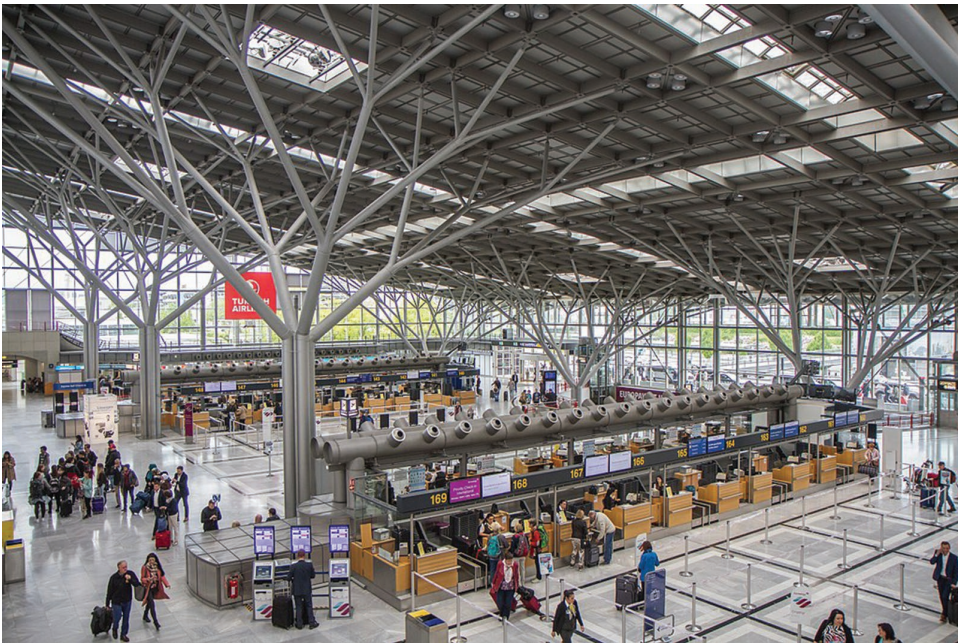
Figure 24.6 Tree-like fractal beams in Stuttgart airport reduce material use for the same strength
