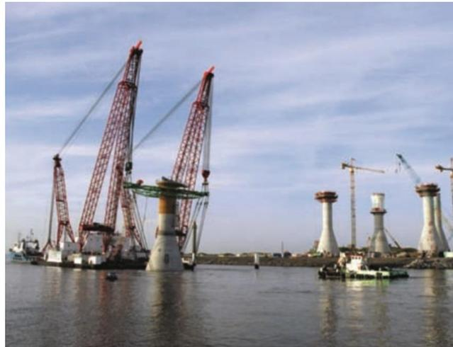
*Figure A-13 - Heavy lift vessel lifting a gravity based foundation
