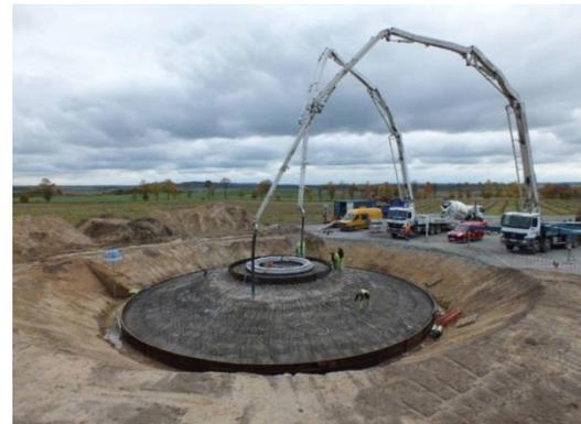
Figure 3-7 - Foundation onshore wind turbine (cte-wind.com)
