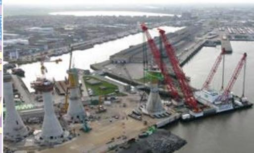
Figure 4-9 - Lifting operation of GBF from the quay wall into the water (c-power.be)
