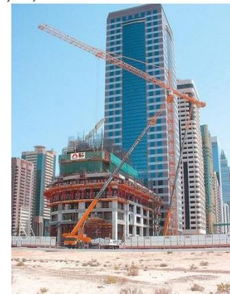
Figure 2-7 - Crane-climbing formwork (peri-usa.com)
