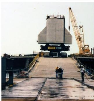
Figure 2-1 - Use of caisson as bridge pier ([severnbridges.org](http://severnbridges.org))
