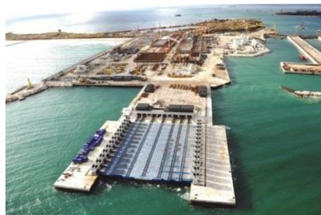
Figure 2-18 – Syncrolift used to transport the caissons into the water (newcivilengineer.com, 2011)
