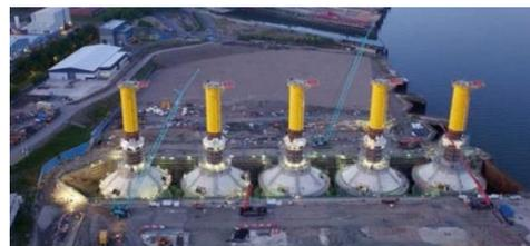
Figure 2-20 - Gravity based foundations for wind turbine in dry dock (bam.com)
