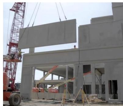
Figure 2-4 - Prefab concrete structure
