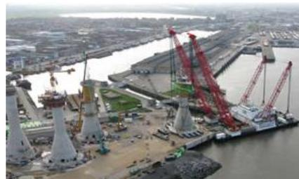
Figure 2-16 - Lifting GBF with the heavy lift barge Rambiz (c-power.be)
