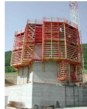
Figure 2-8 - Self-climbing formwork at bridge of Millau (engineersireland.ie)
