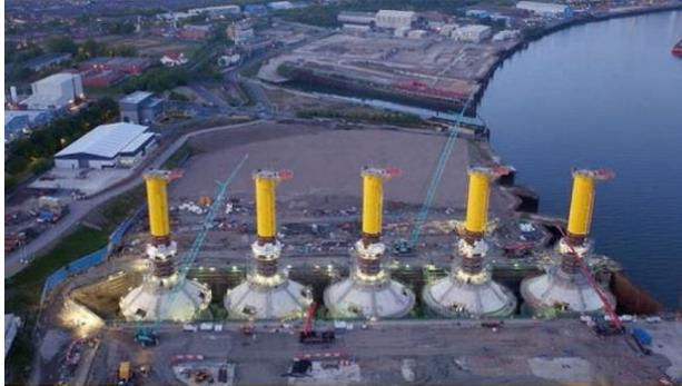
Figure A-7 - Gravity based foundation for wind turbine in dry dock (bam.com)
