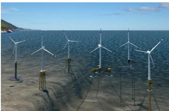
Figure 3-8 - Different types of offshore wind turbine foundations (energy.gov, 2017)
