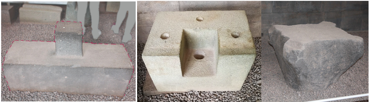
Figures 2.20 and 2.21 demonstrate two examples of the interlocking technique. Images and annotation by author. Figure 2.22 courtesy of Atticus Drake
