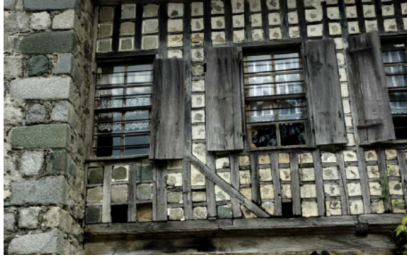
Figures 3.3 and 3.4- Wall cell infill systems. Images by Hamiyet Özen.
