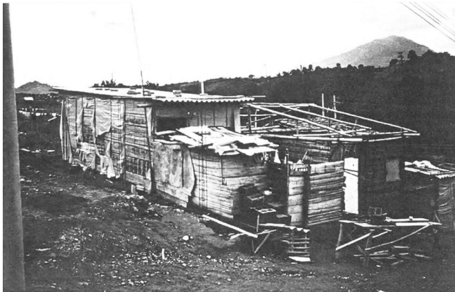
Figure 3.8- Foundations were laid around the outside of a bamboo house in 1992. Image by Katherine Gough
