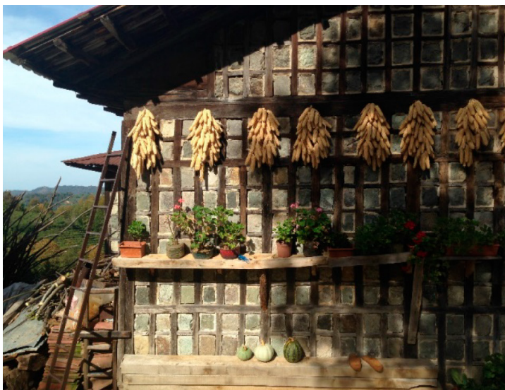
Wooden infill facade system. Photographed by Ömer Faruk Bayram
