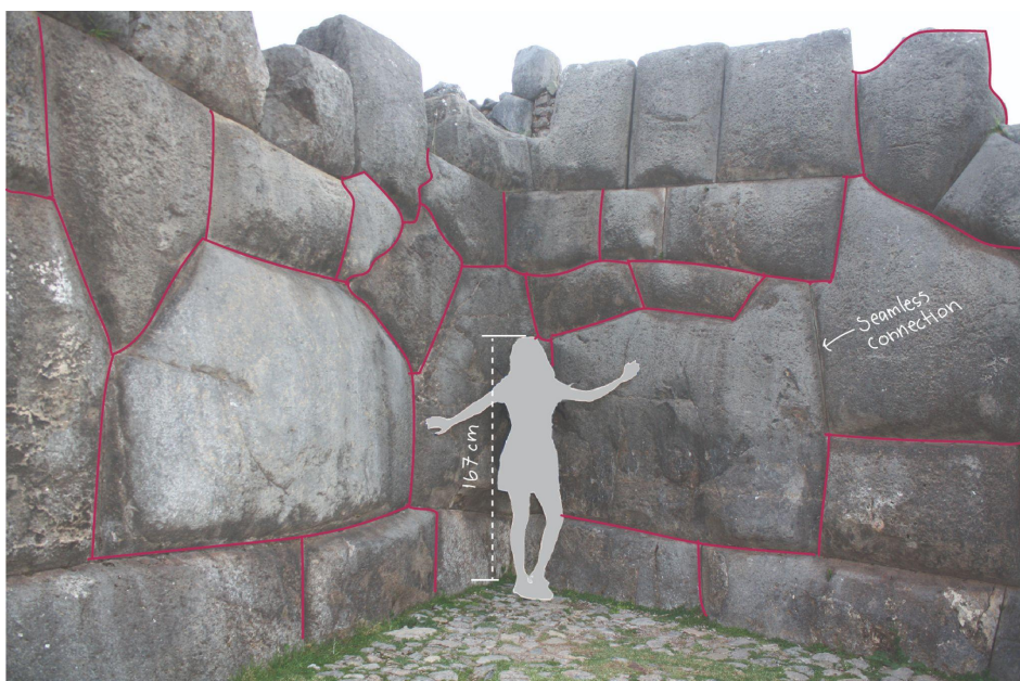
Abuilding corner in Ollantaytambo highlighting the large rock dimensions in reference to human scale. Image and annotation by author
