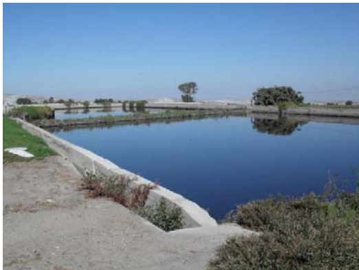
Picture 1 Large Reservoirs at Upstream of Lateral 15
