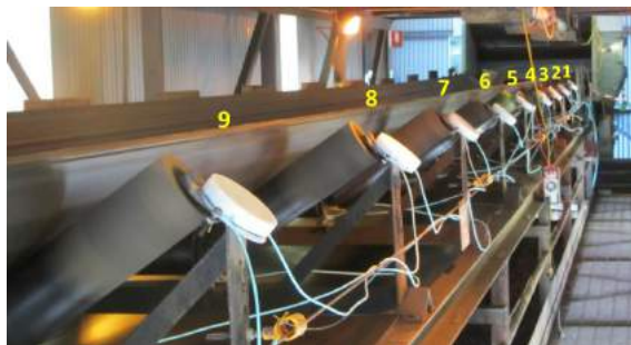
Figure 5.4: Fibre optic-based distributed temperature sensing system, derived from Yang (2014).
