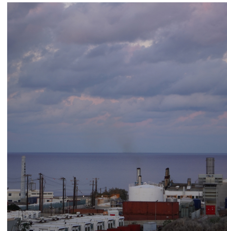
Figure 6. Oil thermal unit
