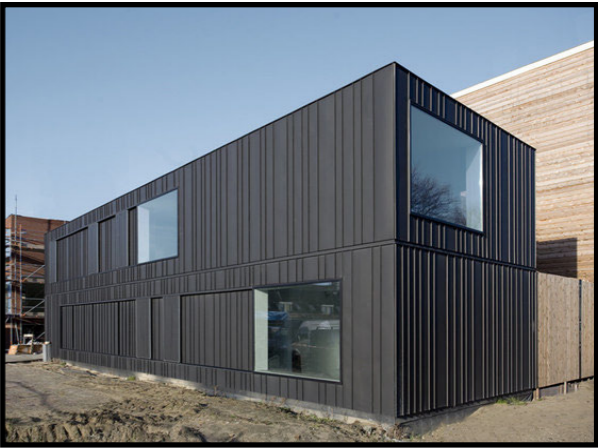
Material - dark pre-patinated zinc PROJECT BY PASEL.KUENZEL ARCHITECTS ROTTERDAM, NETHERLANDS
