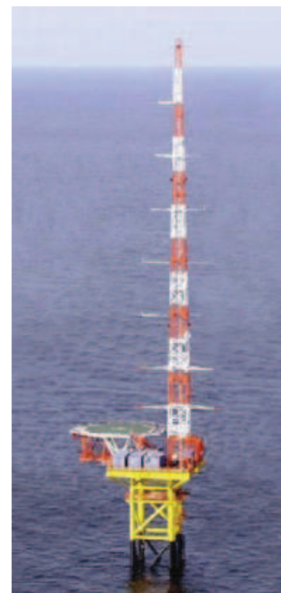
Figure 3.8: FINO1 - Offshore research platform [14]
