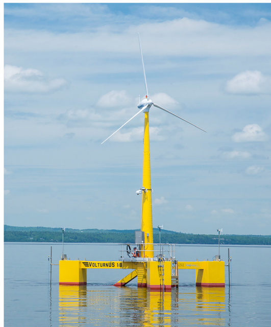
Figure 2.6: VoltturnUS 1:8 model with composite tower [16]
