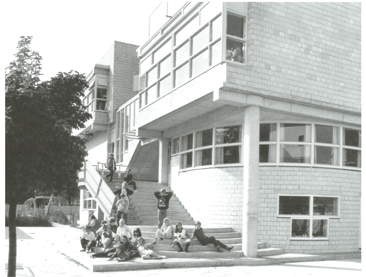
figure 18 - Exterior of Montessorischool - Hertzberger 1980
