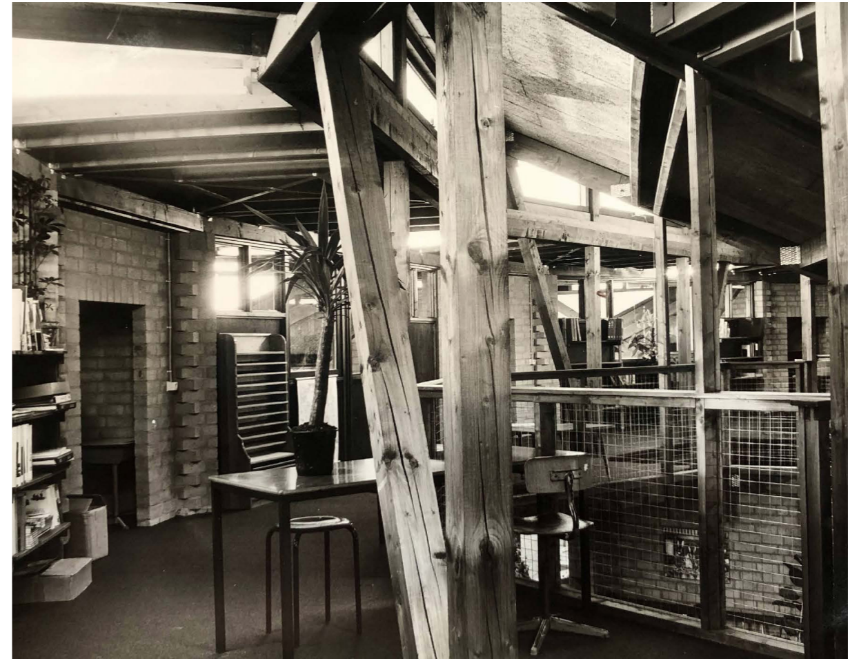
figure 08 - View over balcony, 't Ronde - Verhoeven 1979
