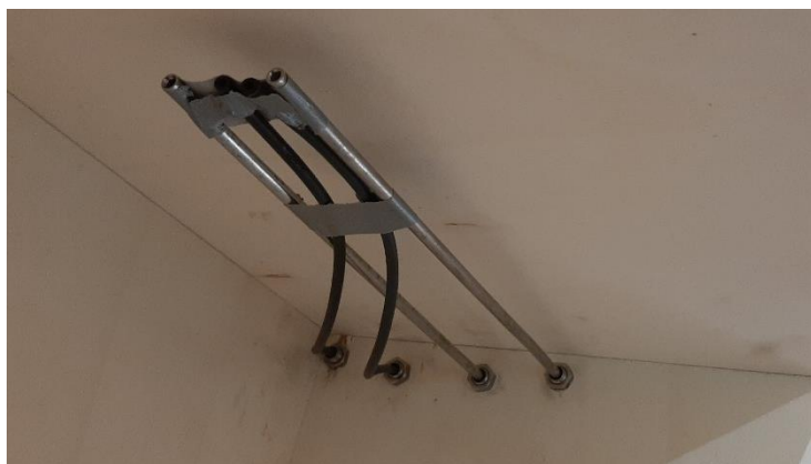
Figure 5-1 Inlets of the 4 (electrochemical) sensors positioned together in one spot in the top center of the metering cabinet.
