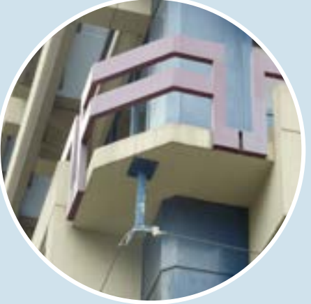
EINDHOVEN POLICE STATION Steel railings Reused for balconies
