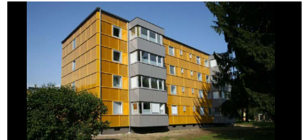
East-block facade renovations energy cost reduction
