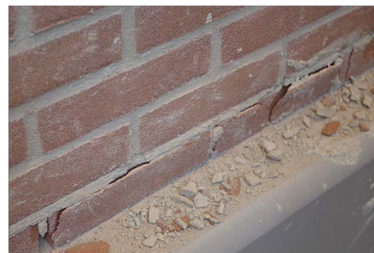
Figure 17 – Crack pattern on the North side: (a) overview; (b) diagonal cracks; (c) diagonal crack top right corner; (d) out-of-plane sliding (marked as “OUT” in figure a); (e) splitting of the bricks in the bottom row.
