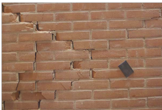
Figure 17 – Crack pattern on the North side: (a) overview; (b) diagonal cracks; (c) diagonal crack top right corner; (d) out-of-plane sliding (marked as “OUT” in figure a); (e) splitting of the bricks in the bottom row.
