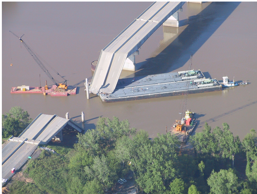
Figure 1.2: The collapsed section of the Interstate 40 bridge, May 31, 2002 [75]
