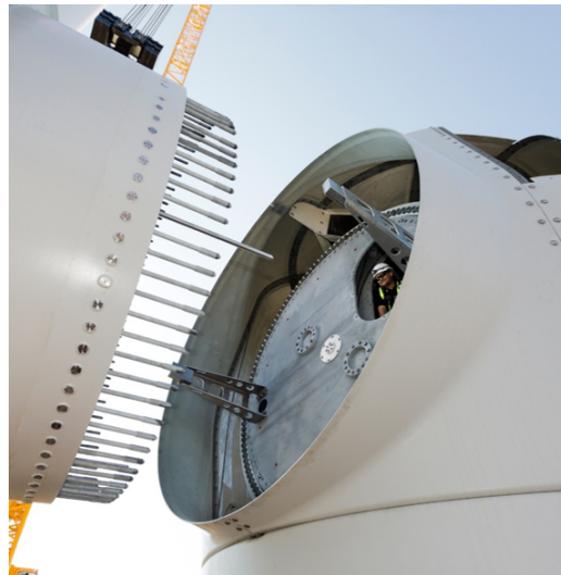
Figure 2.1.2: Connection of a turbine blade to the hub (figure from GustoMSC)
