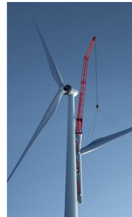
Figure 2.1.8: Climbing crane by Lagerwey [7]
