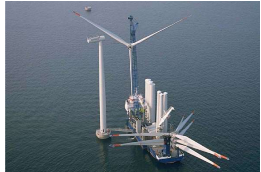
Figure 2.1.5: Three pre-installed blades [4]
