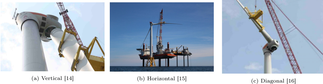
Figure 2.1.3: Single blade installation methods
