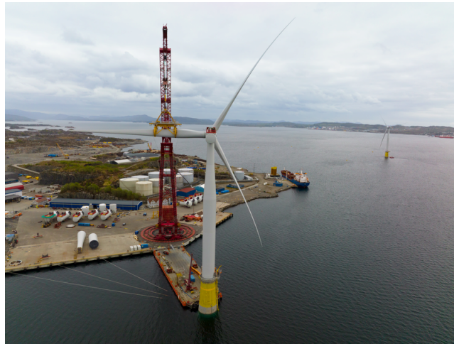
Figure 2.22: Fully assembled spar wind turbine at Wergeland Base, Photo by Jan Arne Wold/Woldcam/Equinor
