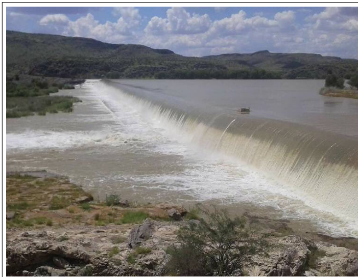
Figure 4.1: Run-of-River weir on the Orange River in South Africa
