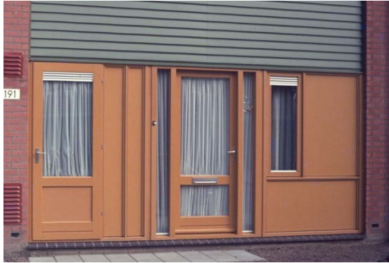
Figure 3, after completion, 1983 (van der Werf, 2017).
