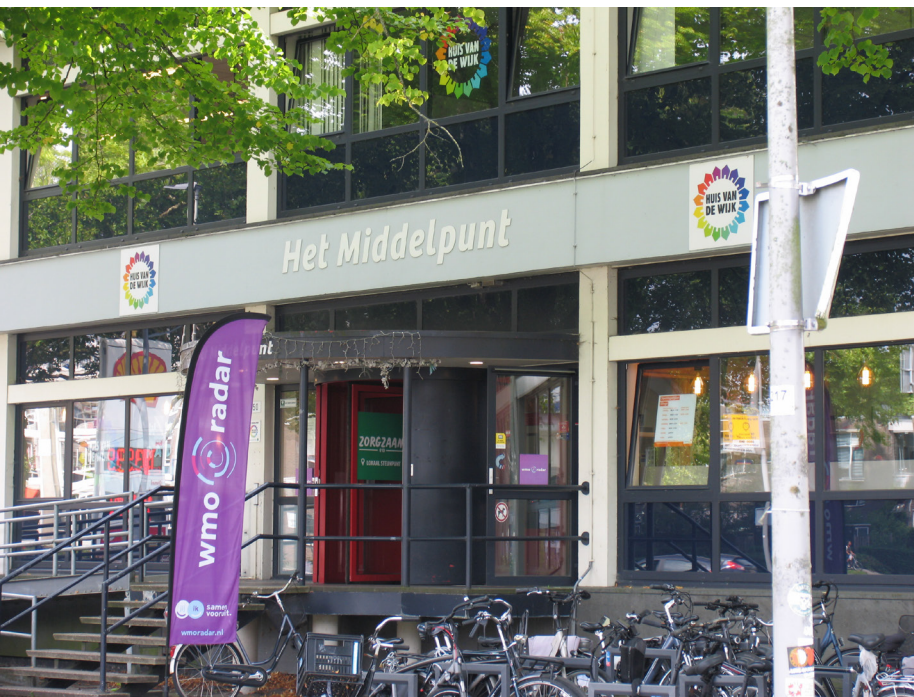
Community centre in Kleinpolder
