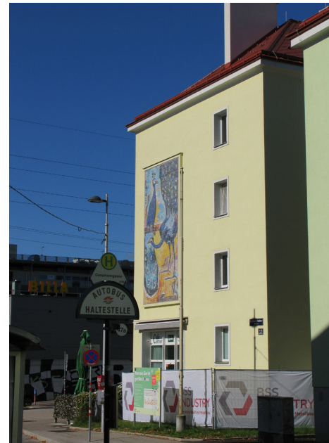
Left: Art windows and entrance on otherwise in-active side façade in Hugo-Breitner-Hof. Below: Balcony's, entrances and art in Jedleseestraße.
