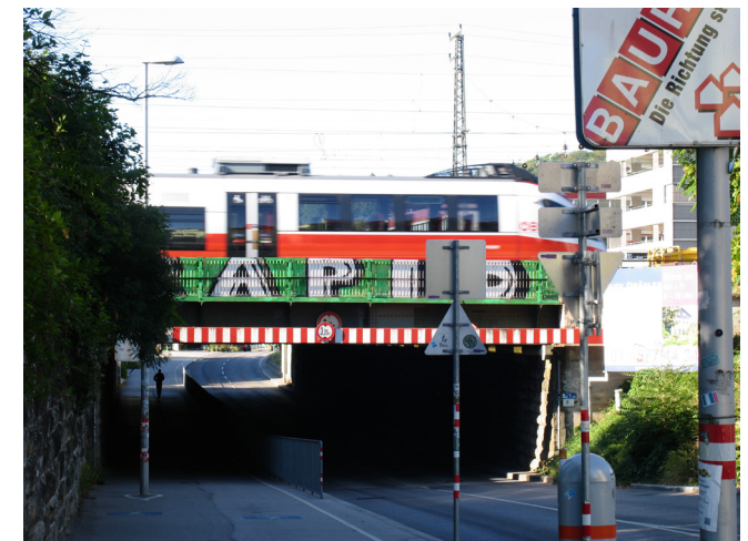
Right: Railway to Hütteldorf Bahnhof as seen from the Hugo-Breitner-Hof Source: Photo by author.
