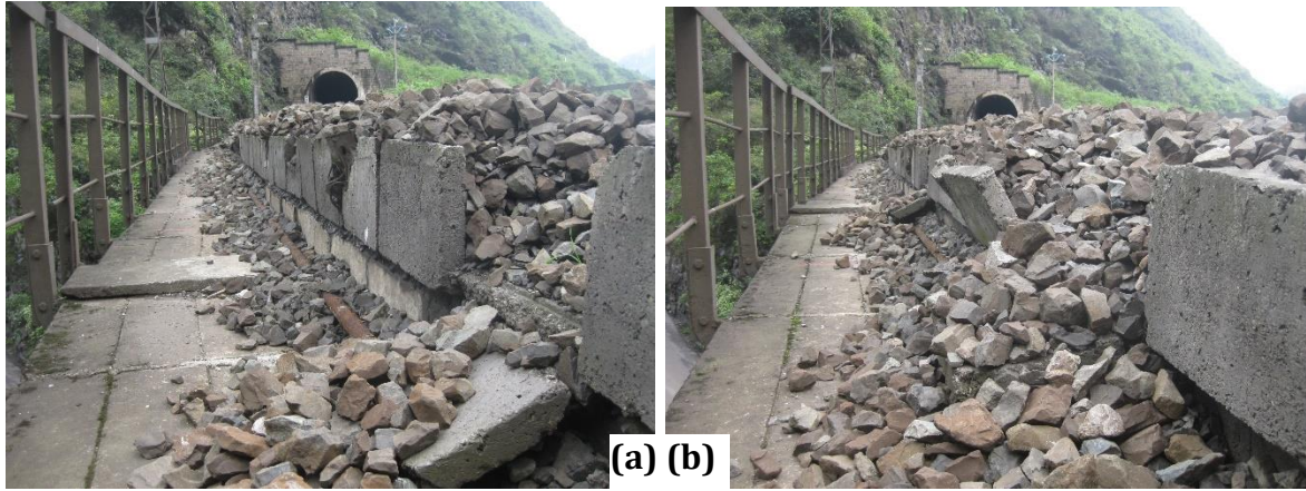
67 Fig. 2 Side view of ballasted track on a bridge with (a) partial damage (b) complete collapse of retaining walls.
