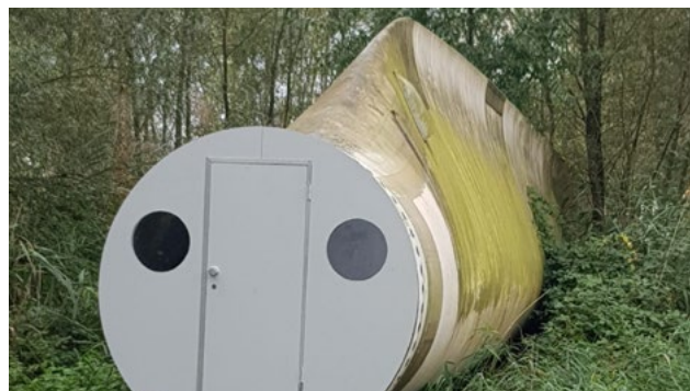
Figure 3.18. Observation of biological growth on wind turbine
