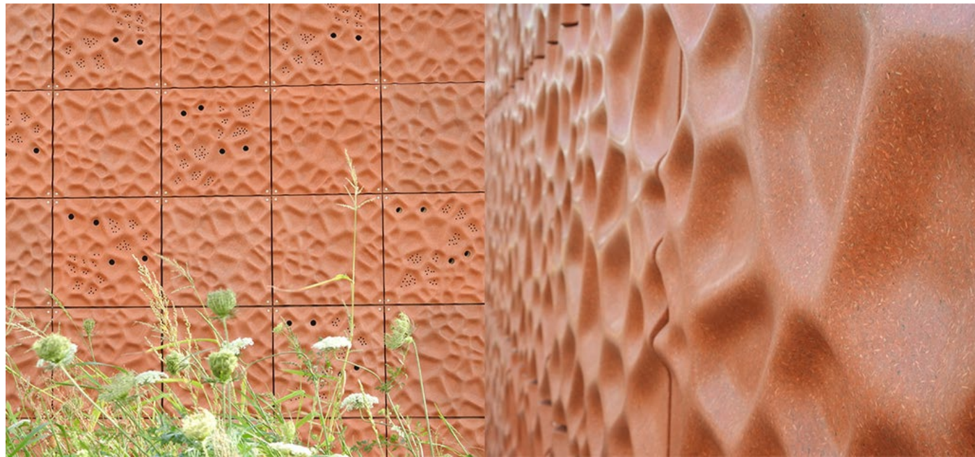
Figure 1.1. Example of a current NPSP facade design using polyester resin, including integrated insect hotels and bird nesting features
