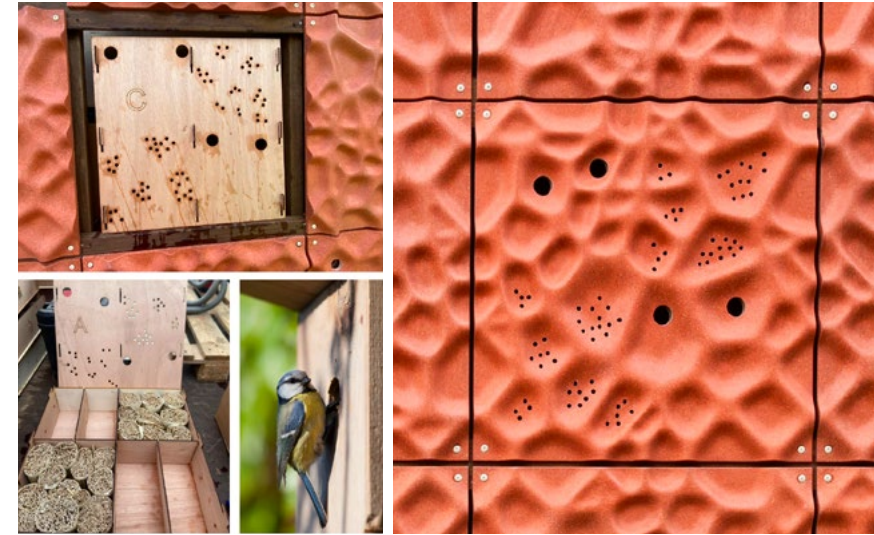
Figure 3.13. Facade panels from NPSP with integrated holes for insect and bird habitats (Source: NPSP, n.d.-a)
