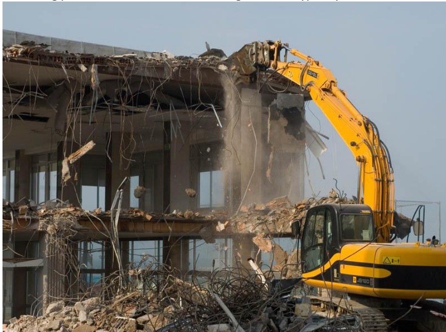
Figure 7; demolishing activities ( http://www.detrez-grondwerken.be/media/images/gallery/20/big/23.jpg )
