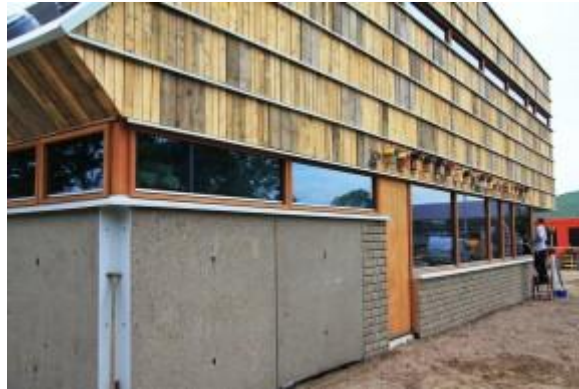
Figure 22; Recycling center Houten, with reused wood and concrete slabs (Bouwwereld.nl)
