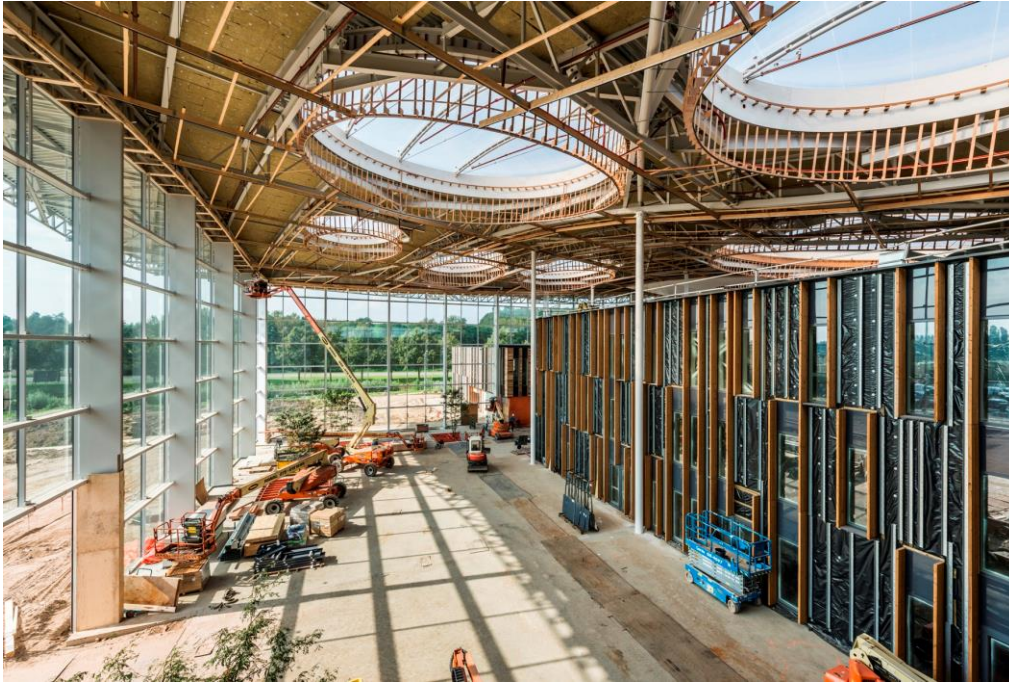
Figure 24; Construction of the roof over the original buildings. The facade on the right is covered with reused wood and insulated with clothing material (Boele.nl)
