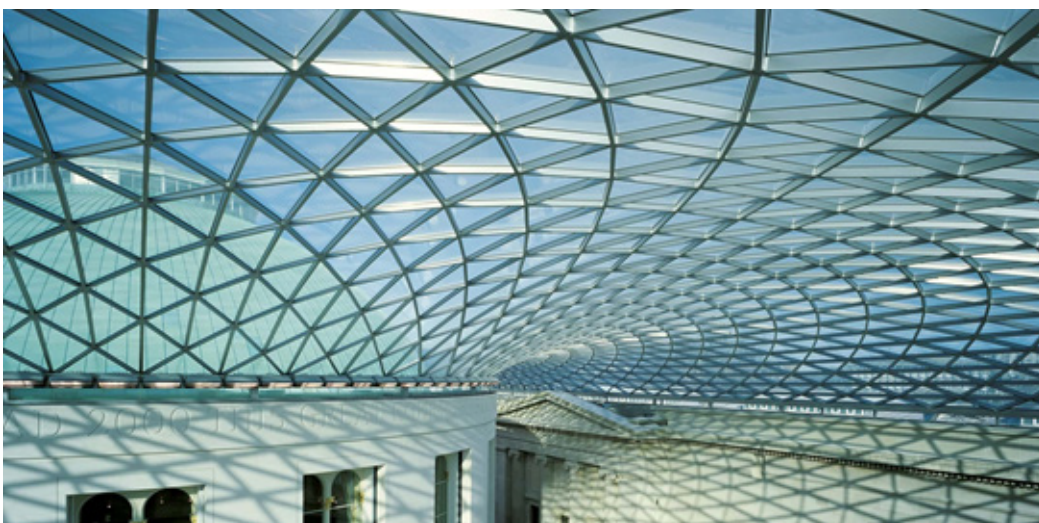
Fig. 3 Lightweight and open: gridshell covering the Queen Elisabeth II Great Court, British Museum, London. Foster and partners
