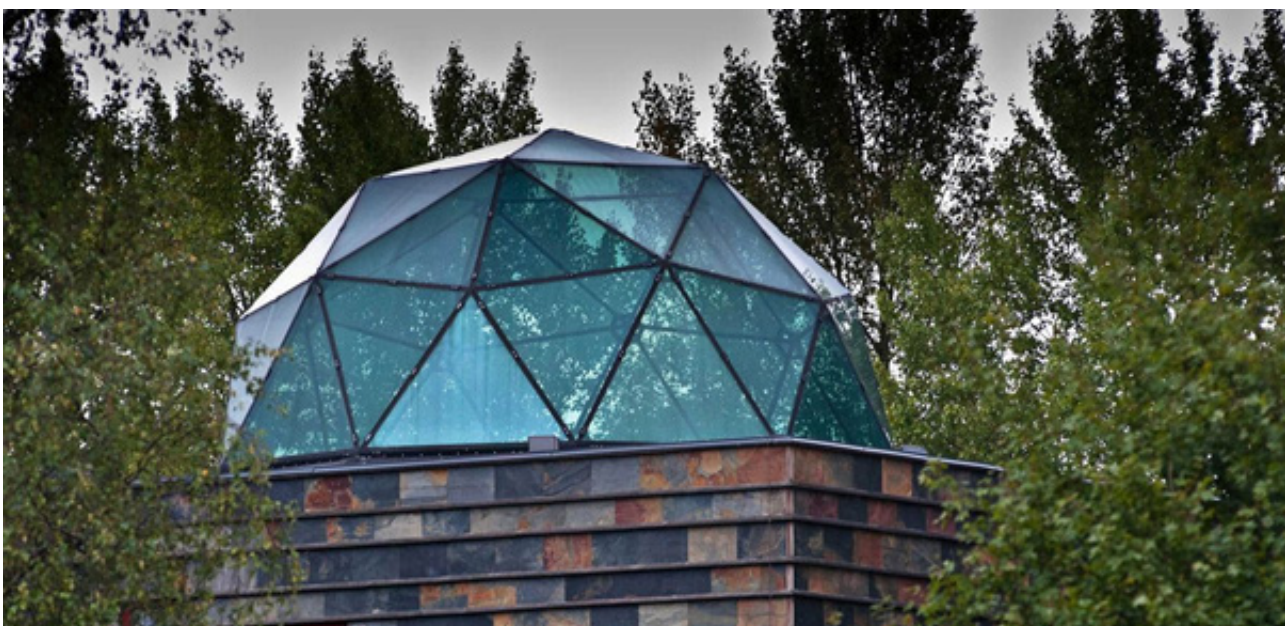
Fig. 66 Pre-tensioned structural glass dome at the Selimiye mosque
