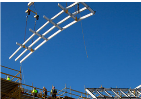
Fig. 38 Simplified on-site assembly using pre-assembled 'ladders'
