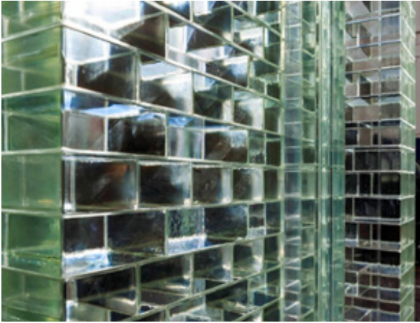
Fig. 121 Detail of the Crystal Houses project, with a 210 x 167.5 x 65 bricks visible at the corner
