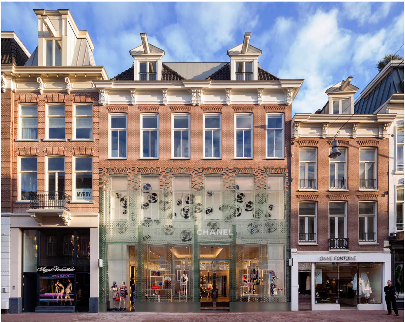
Fig. 15 The finished, part glass brick facade of the Crystal Houses
