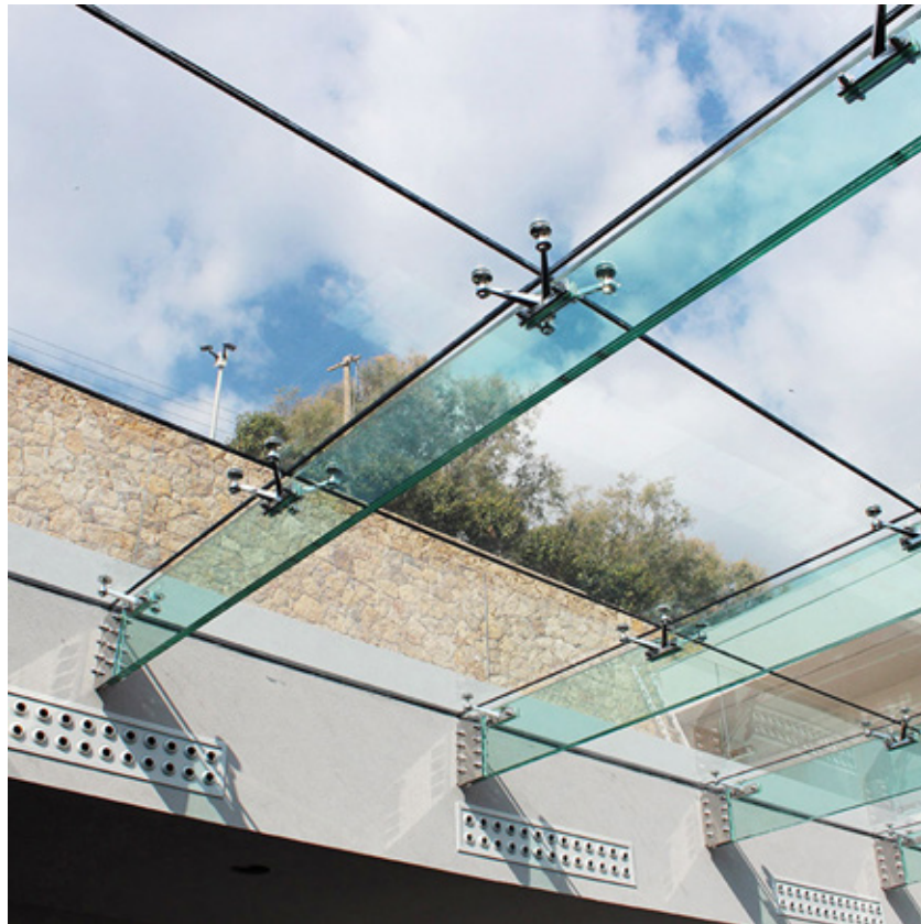
Fig. 56 Example of laminated glass beams
