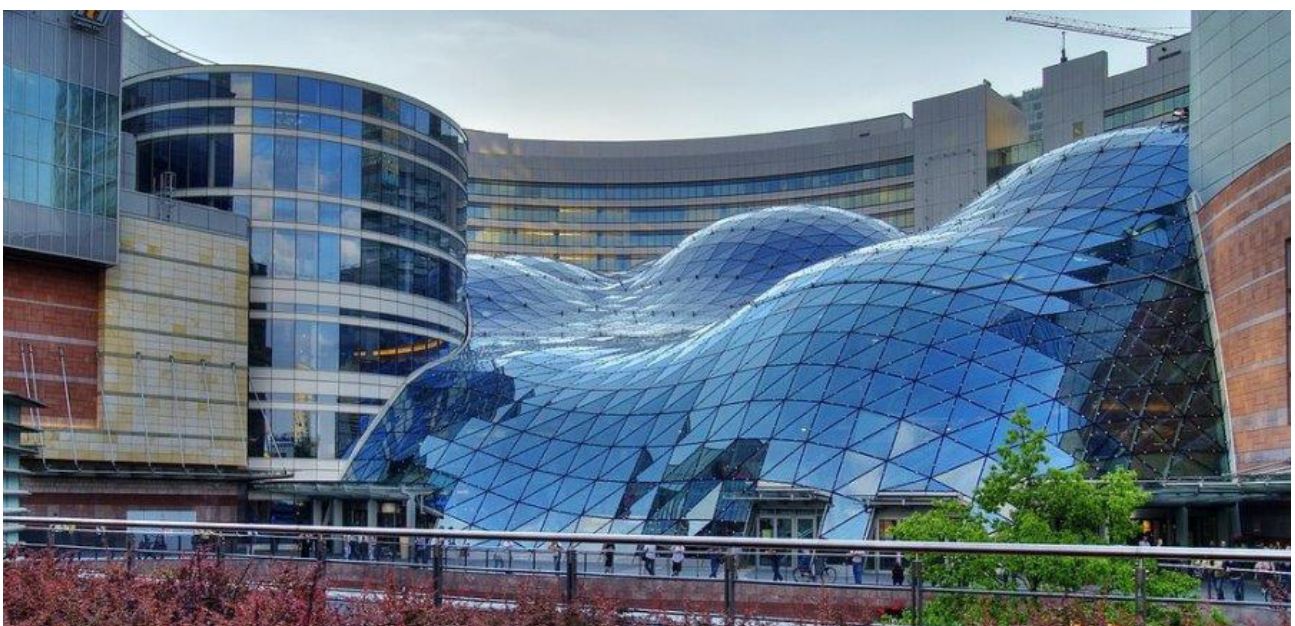
Fig. 105 Gridshell roof of the Złoty Tarasy shopping mall, case study for van der Linden, 2015
