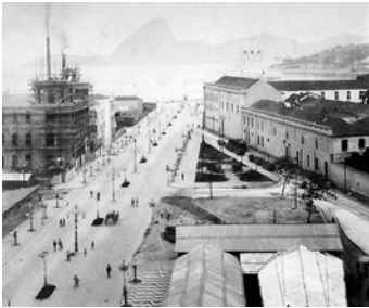
Works in Avenida Central / Avenida Rio Branco, 1905 (source: http://www.flickr.com/photos/11124678@N02/1885274901/in/photostream/ )
