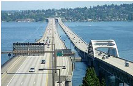
Figure 23: Highway bridge, US
