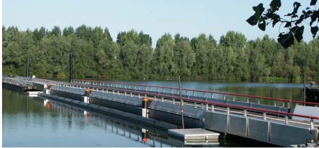
Figure 26: Floating Road, Hedel
