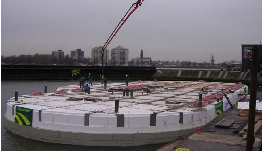
Figure 88: Pouring the beams of the pavilion
