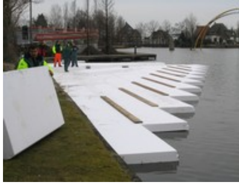
Figure 85: Putting in layer the first layer of EPS, Naaldwijk [Flexbase]
