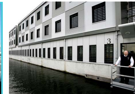
Figure 19: Detention centre, Zaandam
