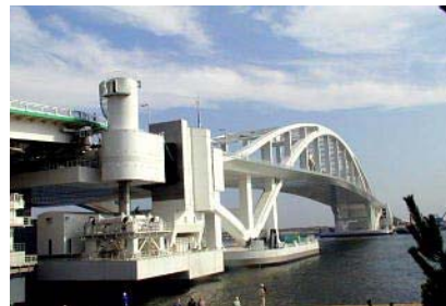
Figure 24: Yumemai Bridge, Japan
