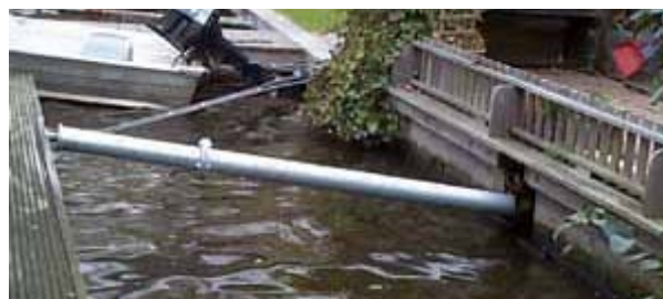
Figure A17-23: Example of Mooring system with rods and cables (ABC Arkenbouw)
