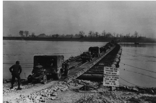
Figure 13: The U.S. 9th Army crosses the Rhine on a temporary steel treadway pontoon bridge, 1945 [wiki]
