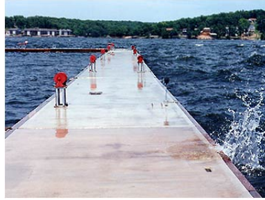
Figure 32: Floating Breakwater, IMF
