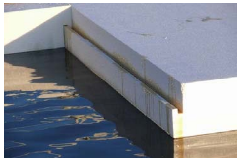
Figure 86: Connecting first layer of EPS with 'haaklas', Greenhouse Naaldwijk [Flexbase]
