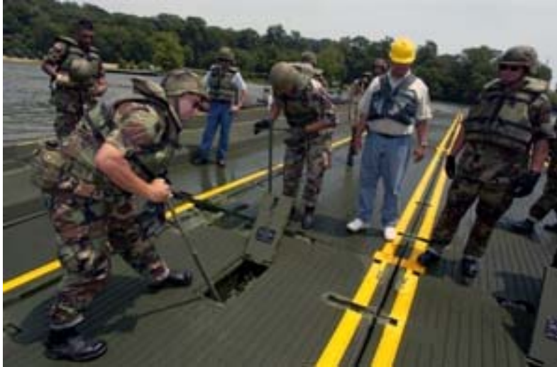
Figure 8: Tightening connection Improved Ribbon Bridge
