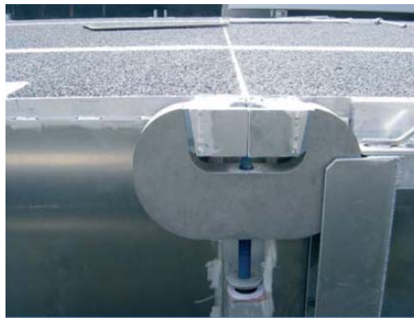
Figure 14: Rigid connection by clamping claw
