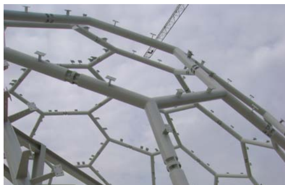
Figure A19-2: Connections superstructure
