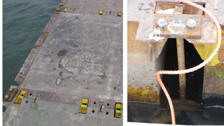
Figure 10: Picture of connection Heijsehaven
