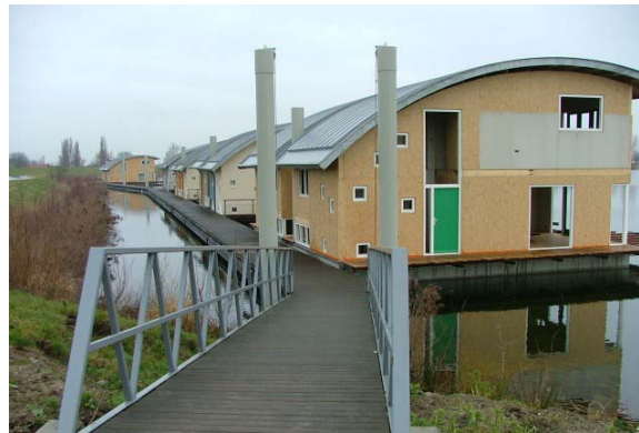
Figure 8: Floating Houses in Maasbommel (Fit, J.J.) ( www.drijvendestad.nl )
