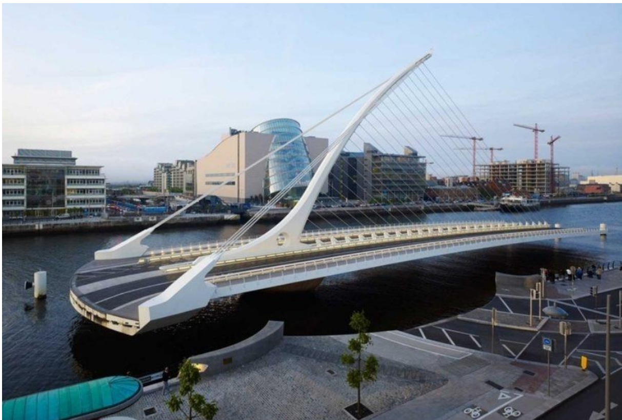
Figure 7.23: Samuel Beckett Bridge in Dublin, opened 2009. A hobsided cable-stayed swingbridge. (Ilovedublin)
