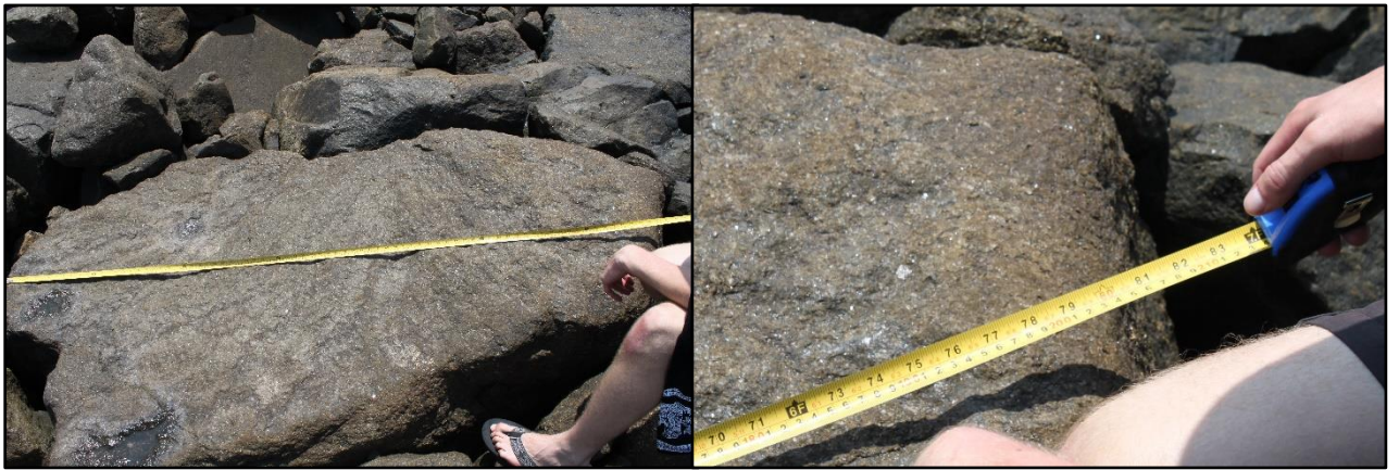
Figure R-4: Armour stone on the breakwater
