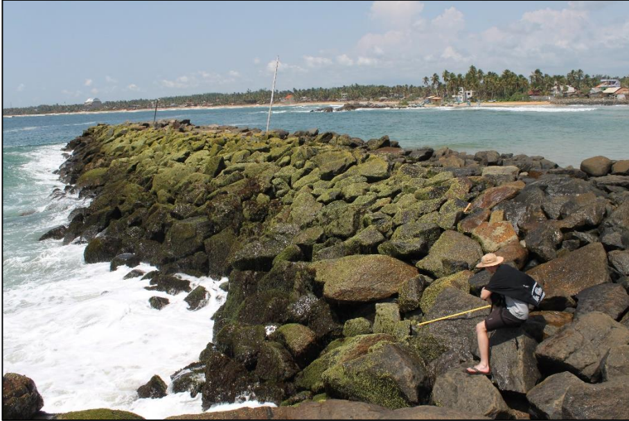
Figure R-22: Measuring stone size current breakwater
