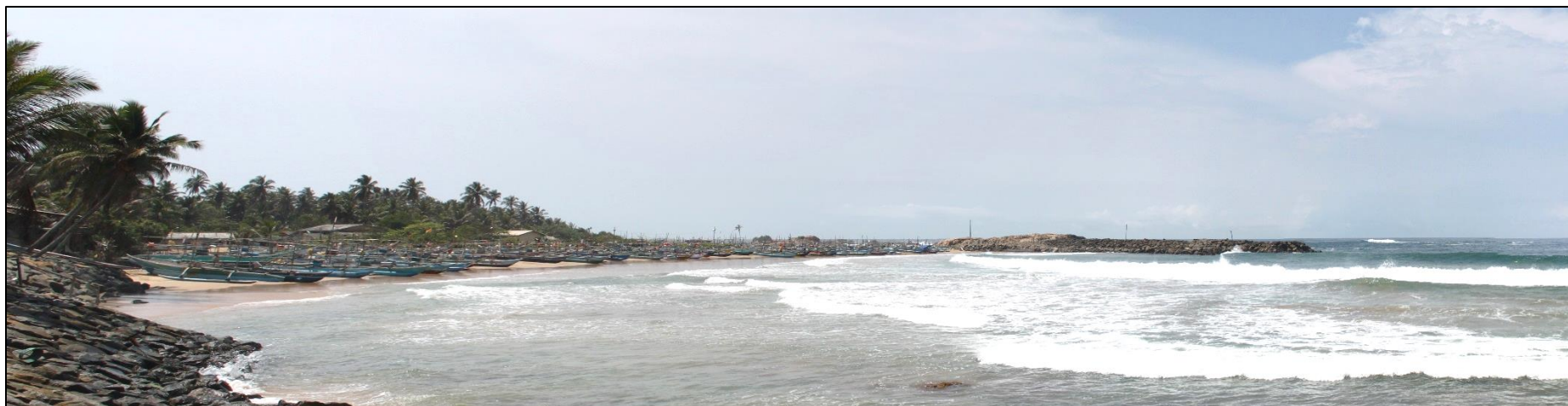
Figure R-19: Panorama photo bay. On the left Vallams, on the right the current breakwater
