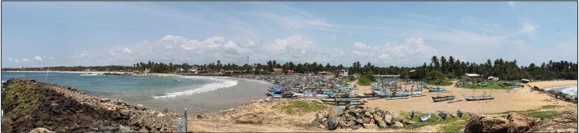
Figure R-21: Panorama photo overview harbour bay
