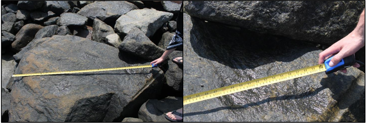
Figure R-3: Armour stone on the breakwater
