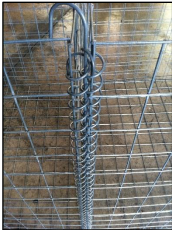
Figure J-6: Spiral connection
