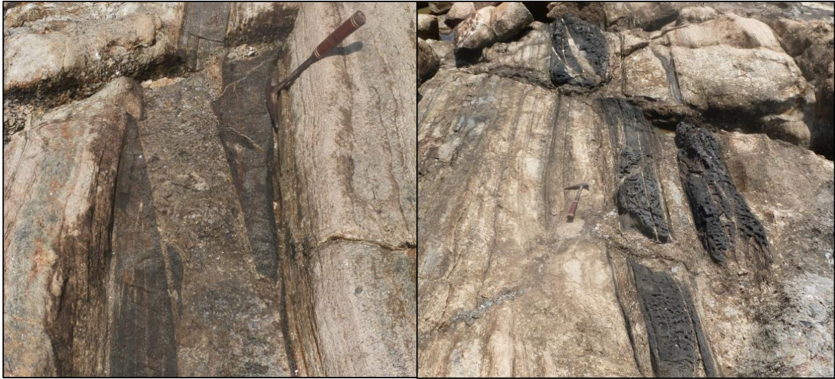
Faults and weathering rocks
