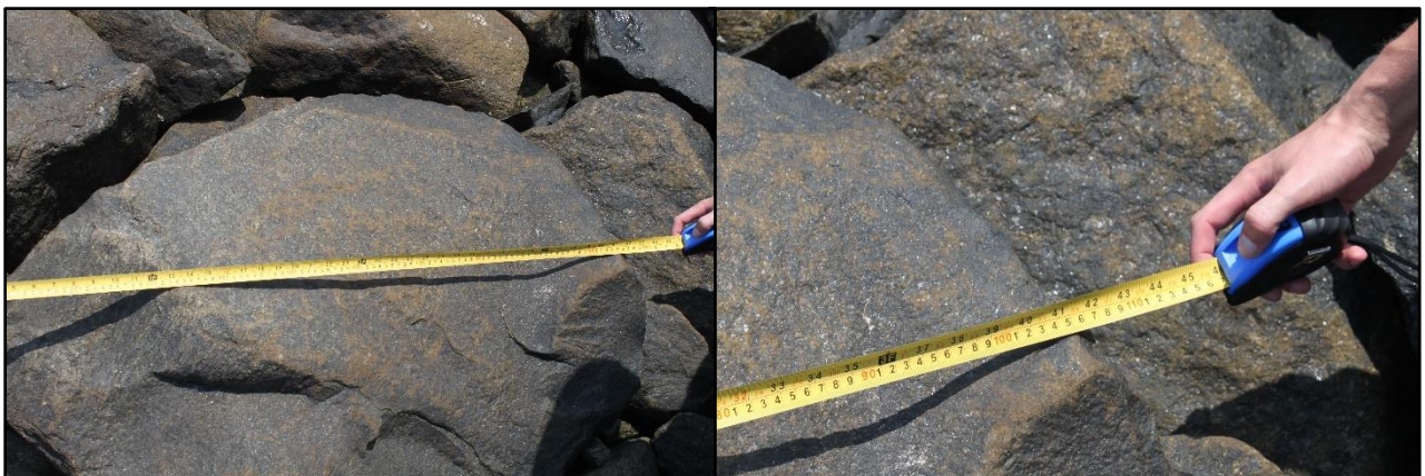
Figure R-2: Armour stone on the breakwater
