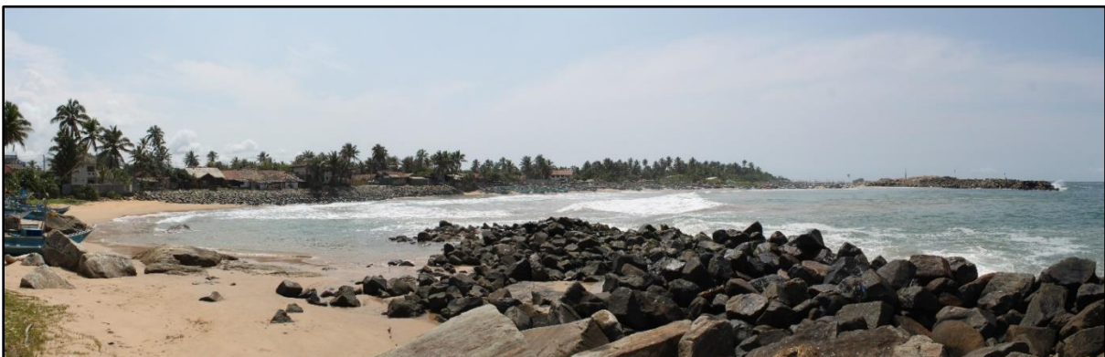
Figure R-6: Armour units extending in the sea
