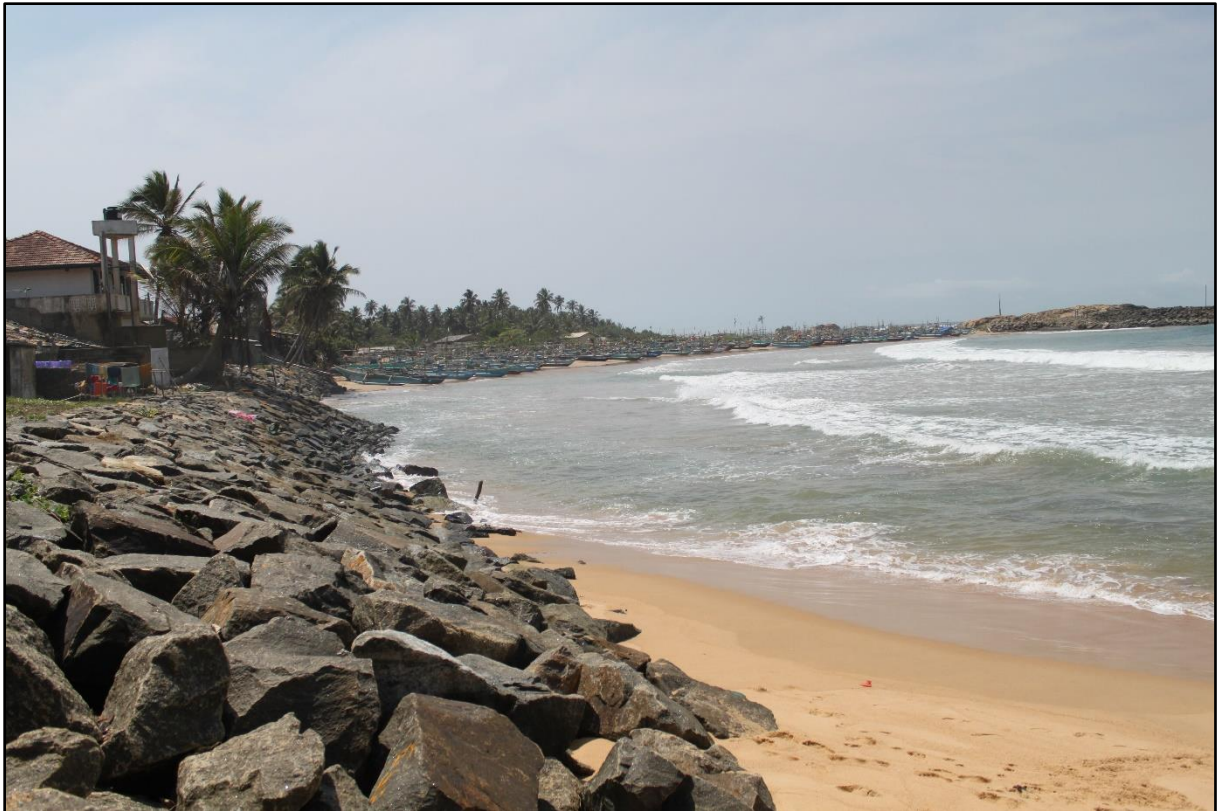
Figure C-7: The revetment in the harbour bay to prevent erosion
