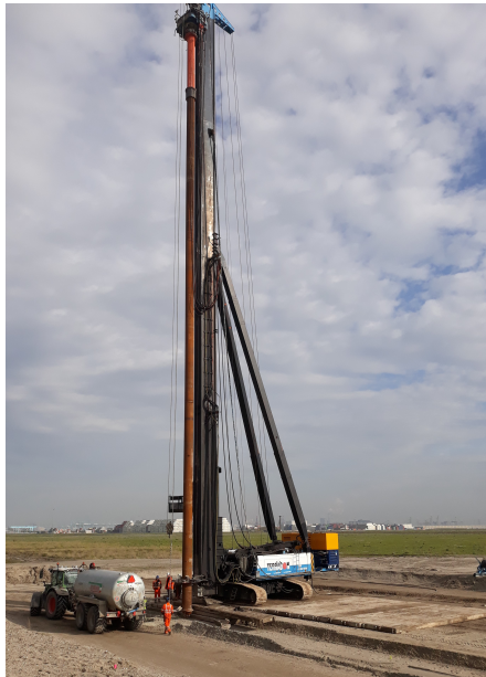
Figure 1.2: Installation of a screw injection pile at the Amaliahaven test site.
