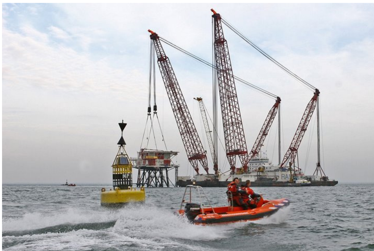
REM island (Noordwijk meetpost Figs. 1.2 and 5.1) in middle of the Rhine ROFI during removal. (image credit: J.A. van Duin).
