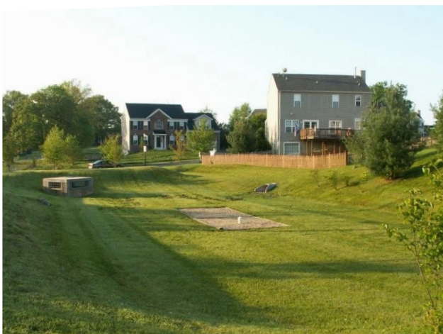
Figure 27. Dry Pond with Sand Filter (www.ecodesigns.com)
