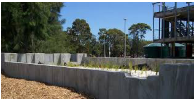
Figure 30. Biofilter at Monash University (Eisenberg and Polcher, 2019)
