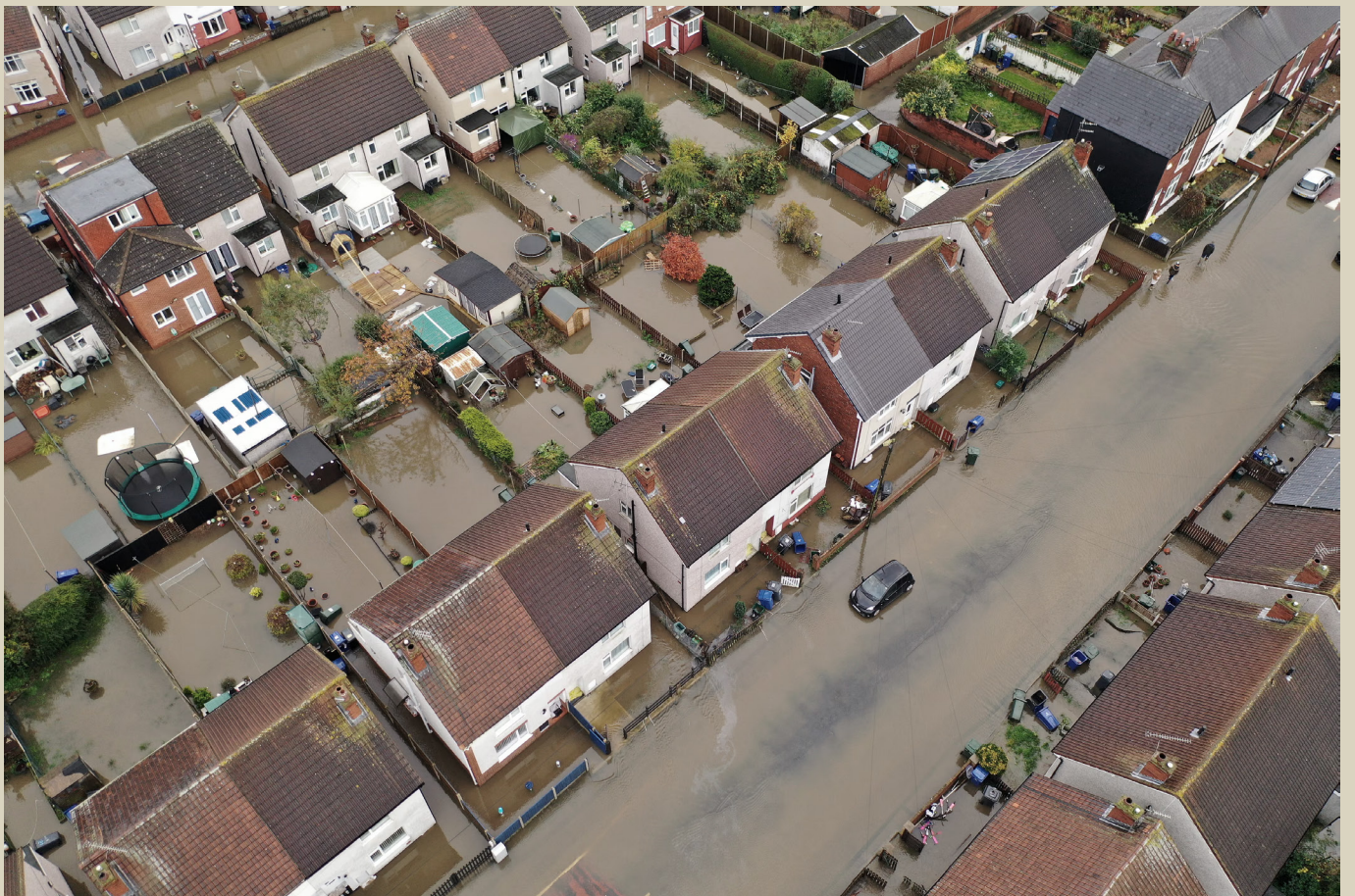
Figure 9. Rainwater inundation entering residential lawns and affecting building surroundings (The Guardian, 2019)
