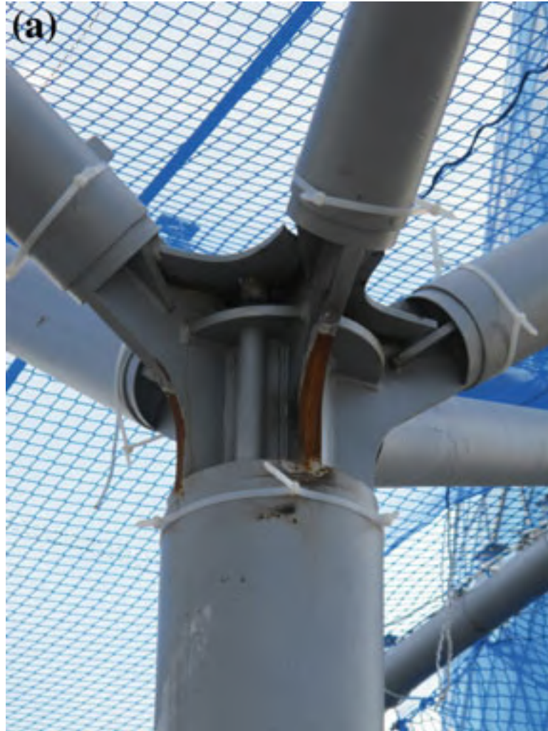
Figure 6.3: Steel plate branched column connection [6.2]
