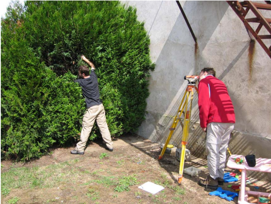
Figure 4-3, Gaining a free line of sight from the levelling instrument to the beacon.
