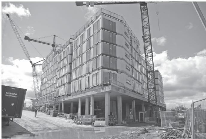
Figure 21 - Modular building with a podium structure (Lawson, Ogden and Goodier 2014)
