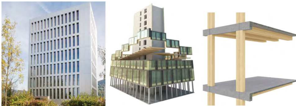
Figure 13 - Life Cycle Tower, prefabricated floor slabs and facade elements (Will+Perkins 2014)
