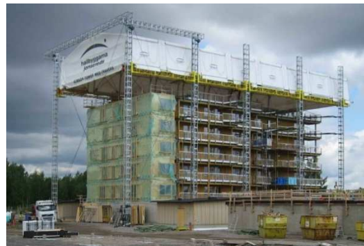
Figure 12 - Limnologen block with weather protection system (Serrano 2009)
