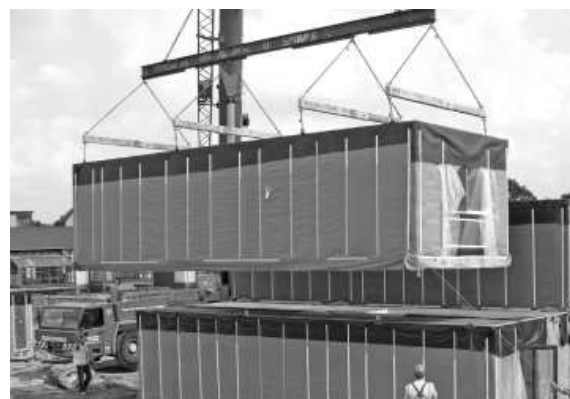
Figure 26 - Lifting of module by main beam and crossbeams (M. Lawson 2014)
