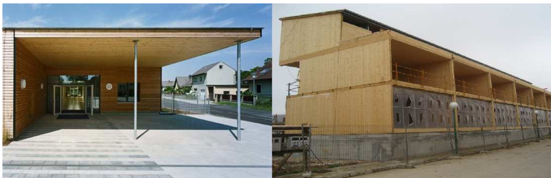
Figure 34 - Point supported CLT panels (left) and line supported CLT panels (right) (Brandner and Schickhofer 2014)
