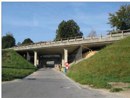
Fig. 6. Slab bridge strengthened with R-UHPFRC over piers (dark areas) in the Switzerland [60].
