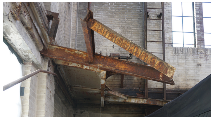
Image 14: Traces of the ovens; a curved hole in the steel construction of the entresol. Source: Luyckx, S.L., 2019.
