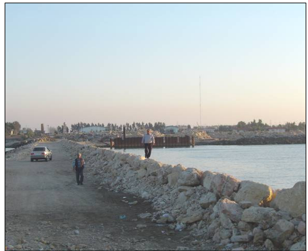
Figure 2-7: Construction of East Breakwater
