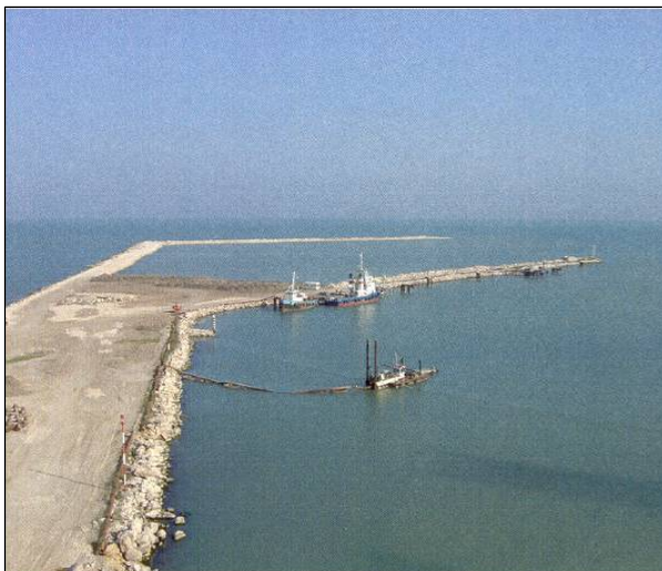
Figure 2-6: Extension of the West Breakwater
