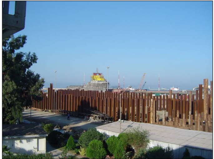
Figure 2-4: Dry Dock under construction
