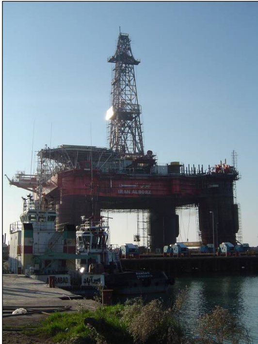
Figure 2-5: Semi Submersible under construction
