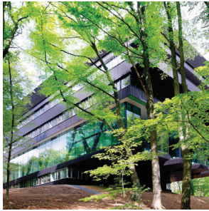
Rehabilitation Centre Groot Klimmendaal, Arnhem, Area: 14,000m 2
